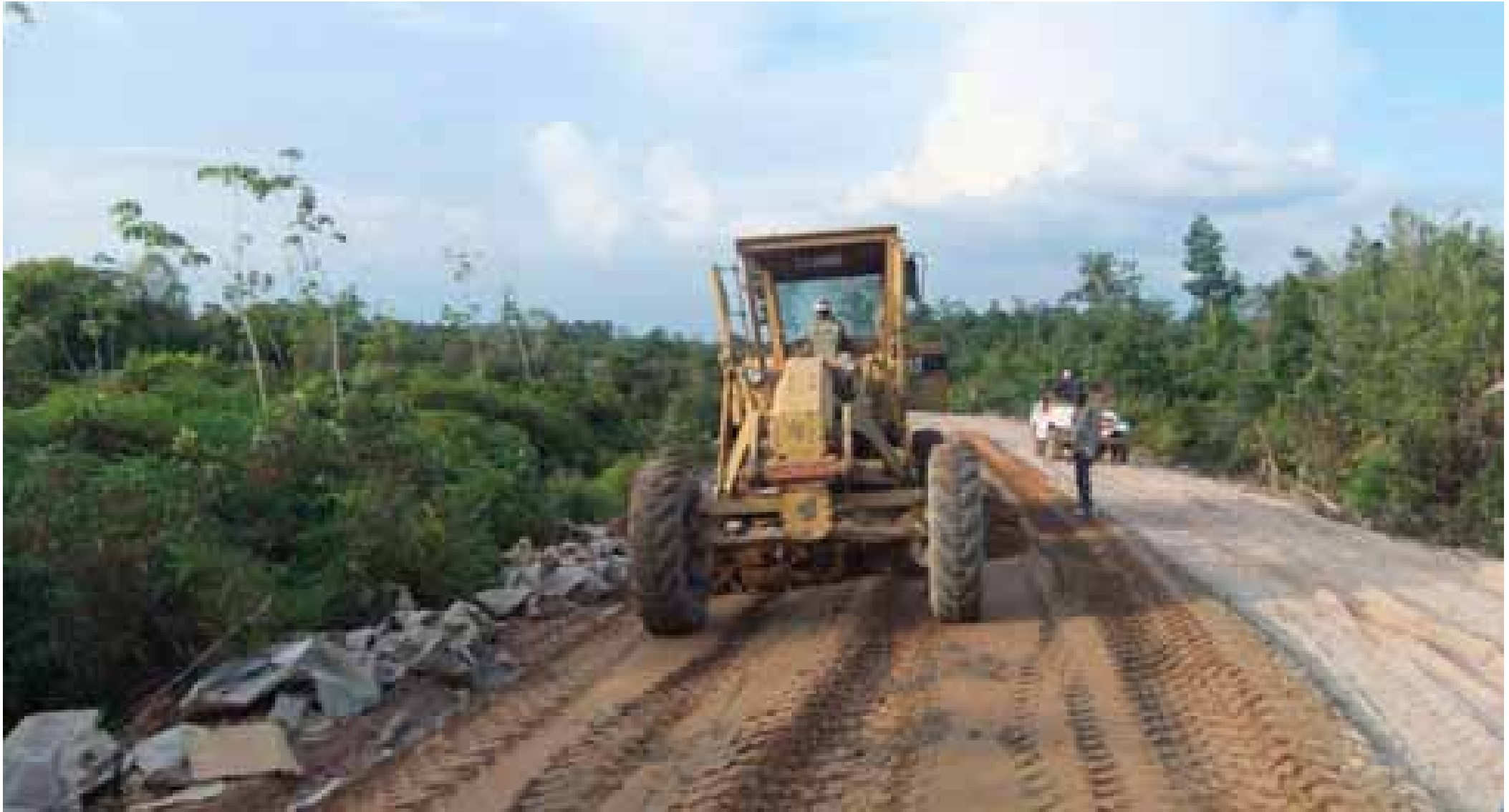
Levelling of the area with a grader
