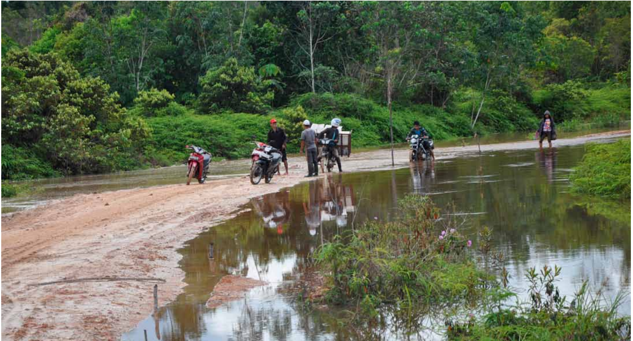
Initial situation after heavy rainfall
