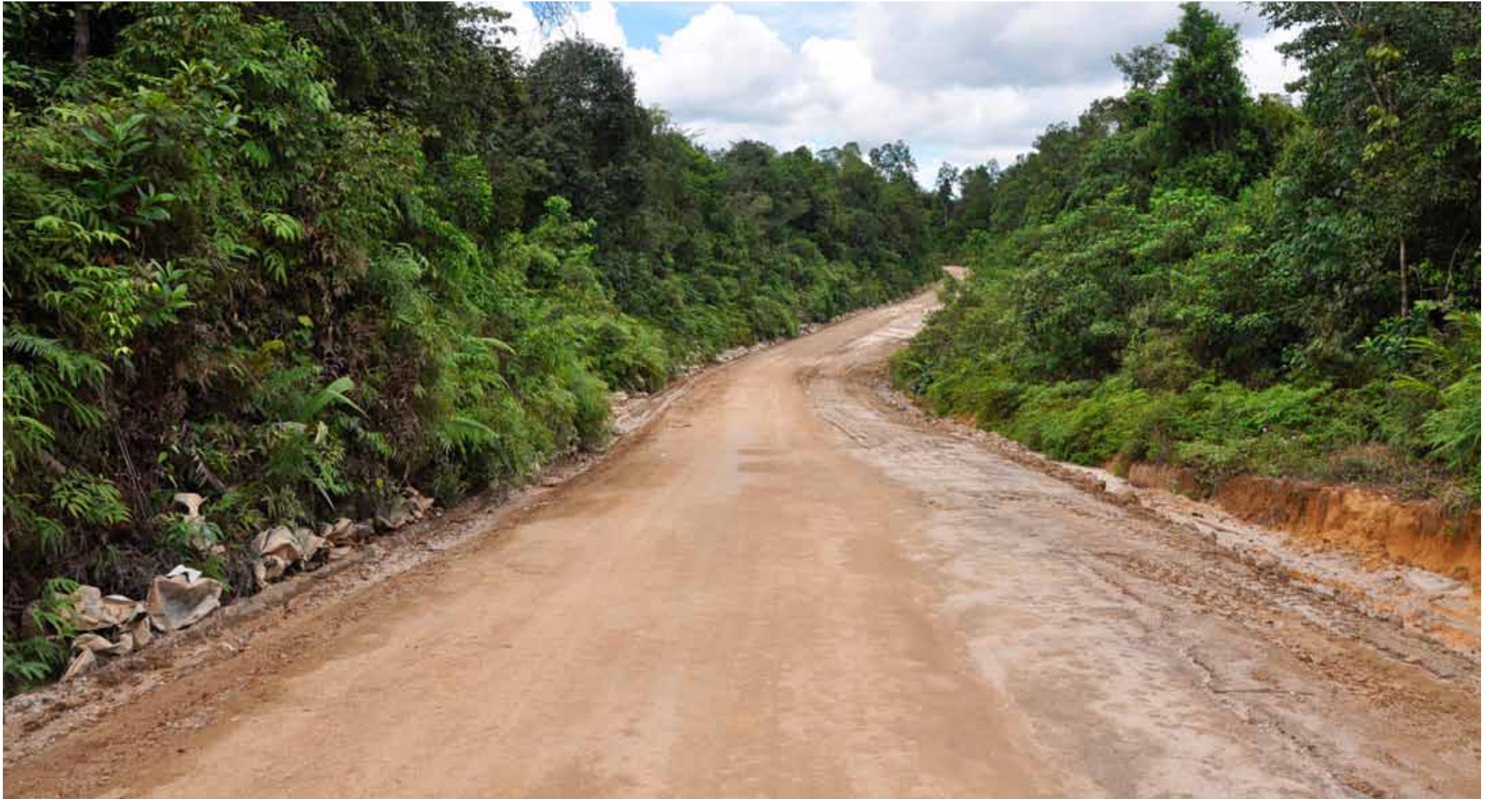
One lane of the finished road
