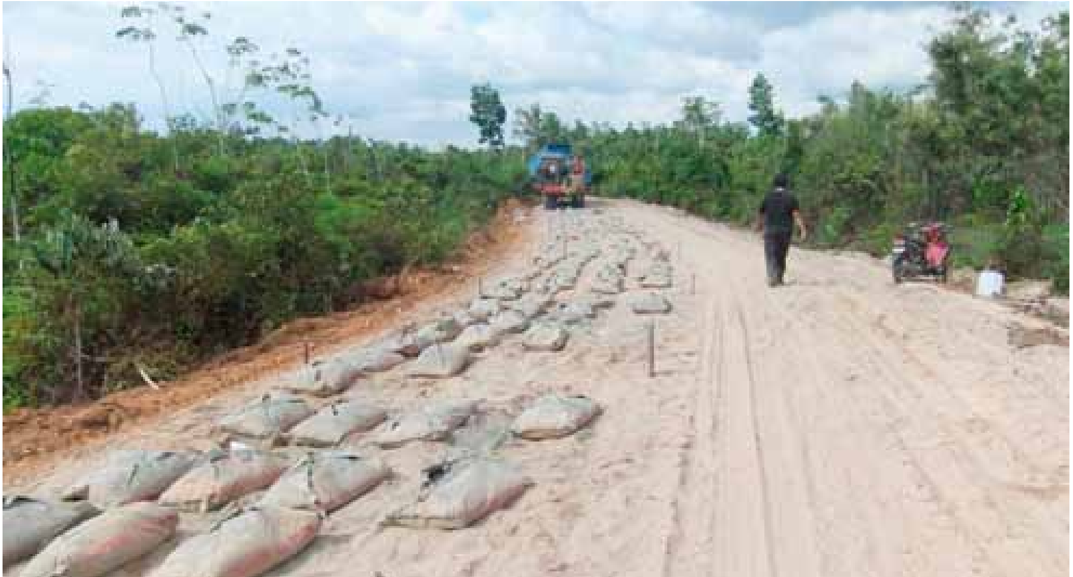
Distribution of the cement bags
