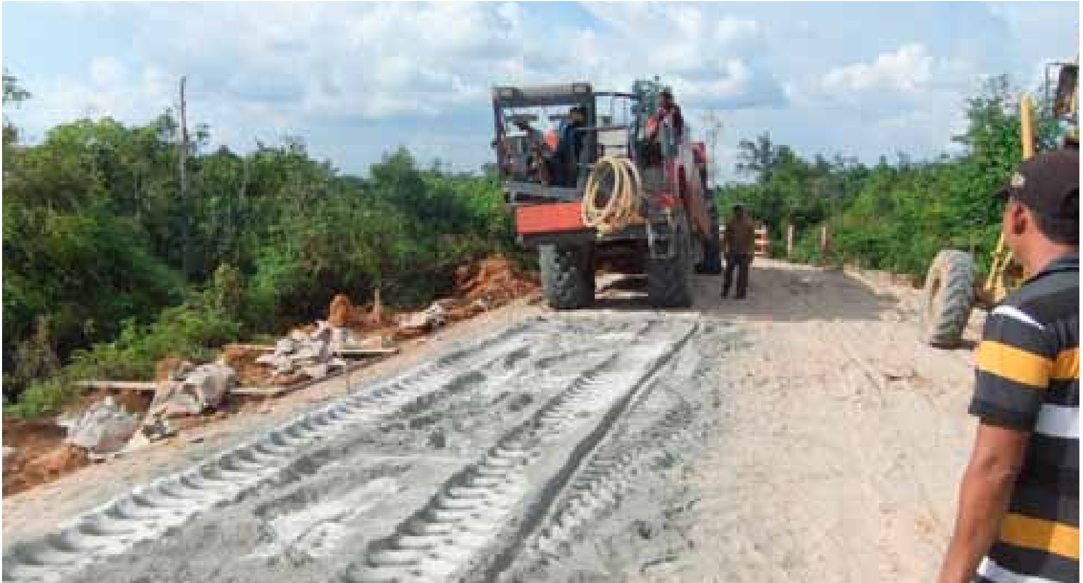
Milling of the cement-Novocrete® mixture up to a depth of 35 cm
