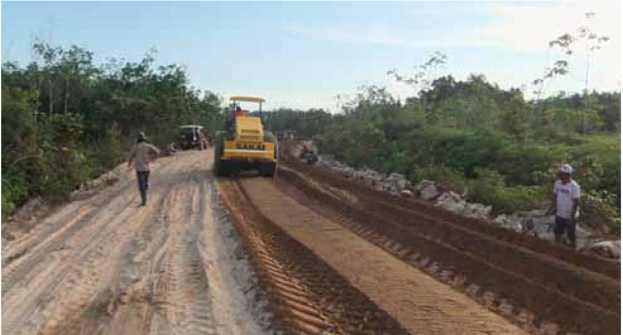
Static and dynamic compaction of the area
