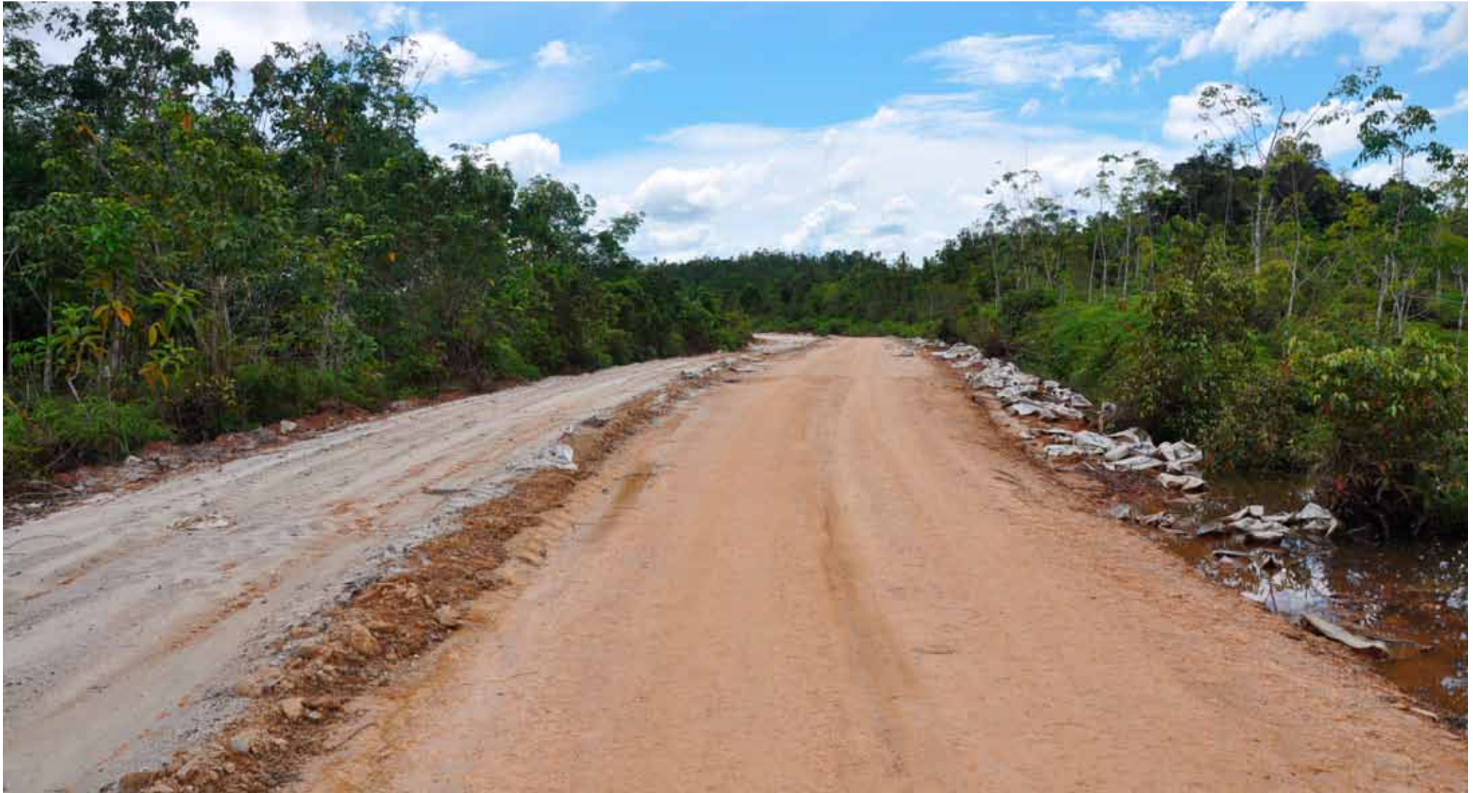
One lane of the finished road
