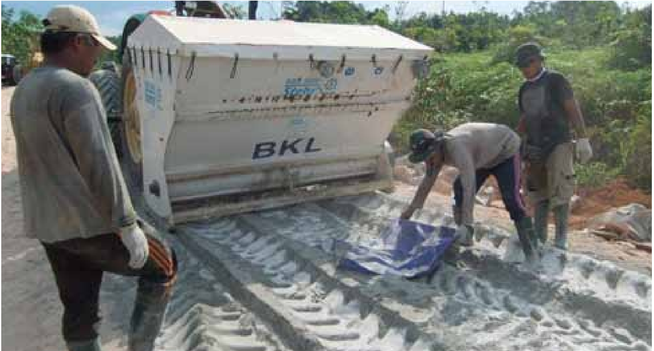
Check of the spreaded amount of NovoCrete®
