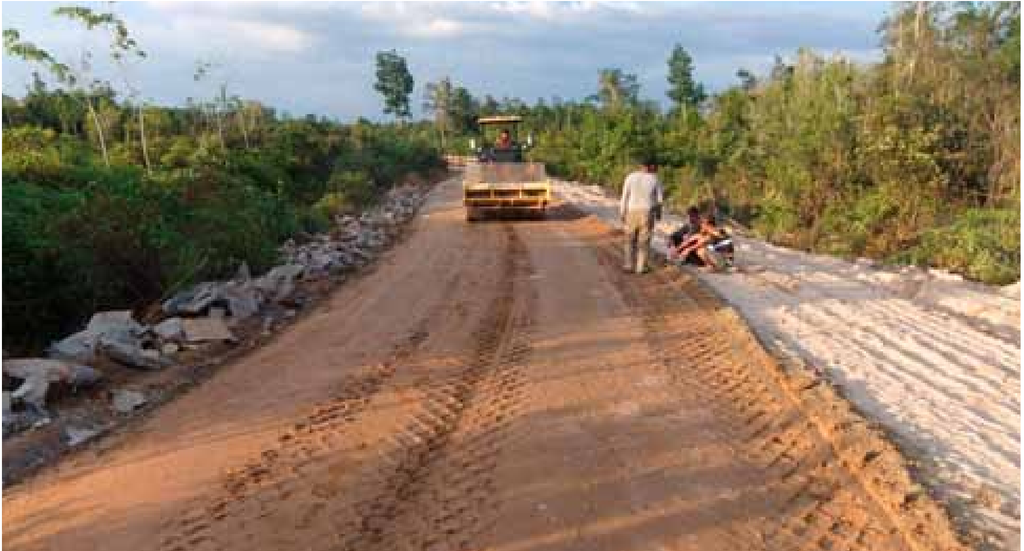
Static and dynamic compaction of the area
