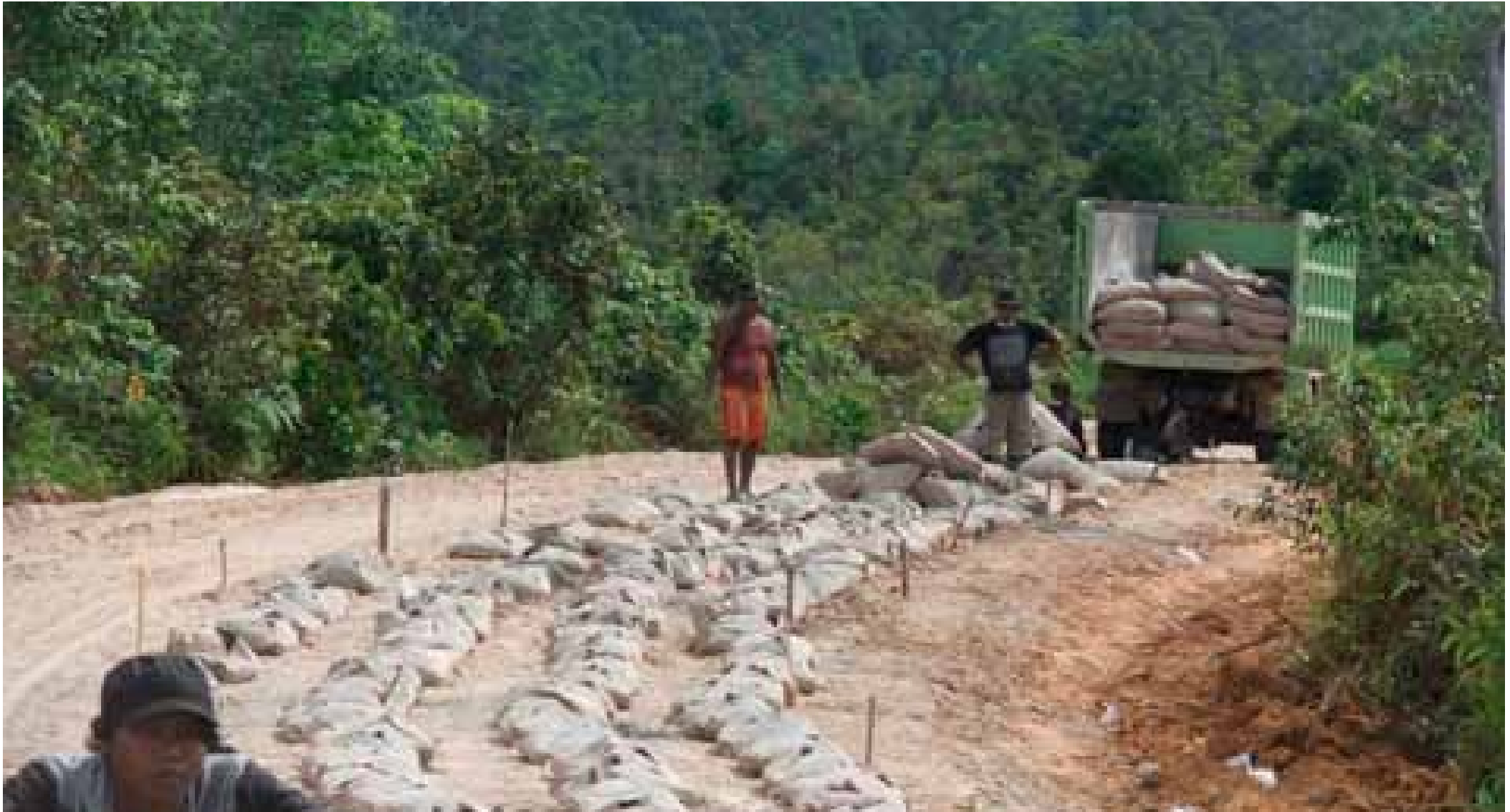
Distribution of the cement bags
