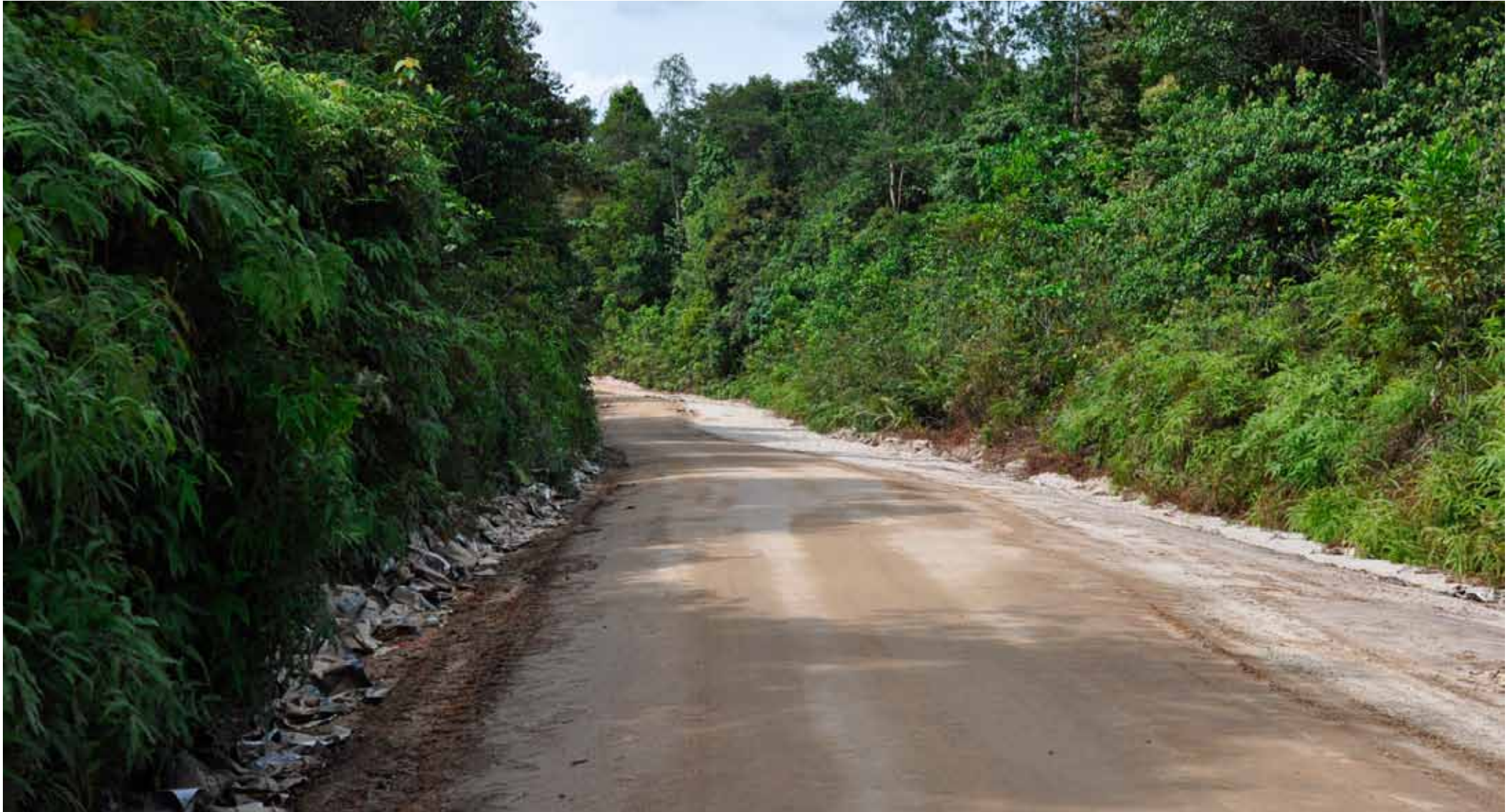
One lane of the finished road
