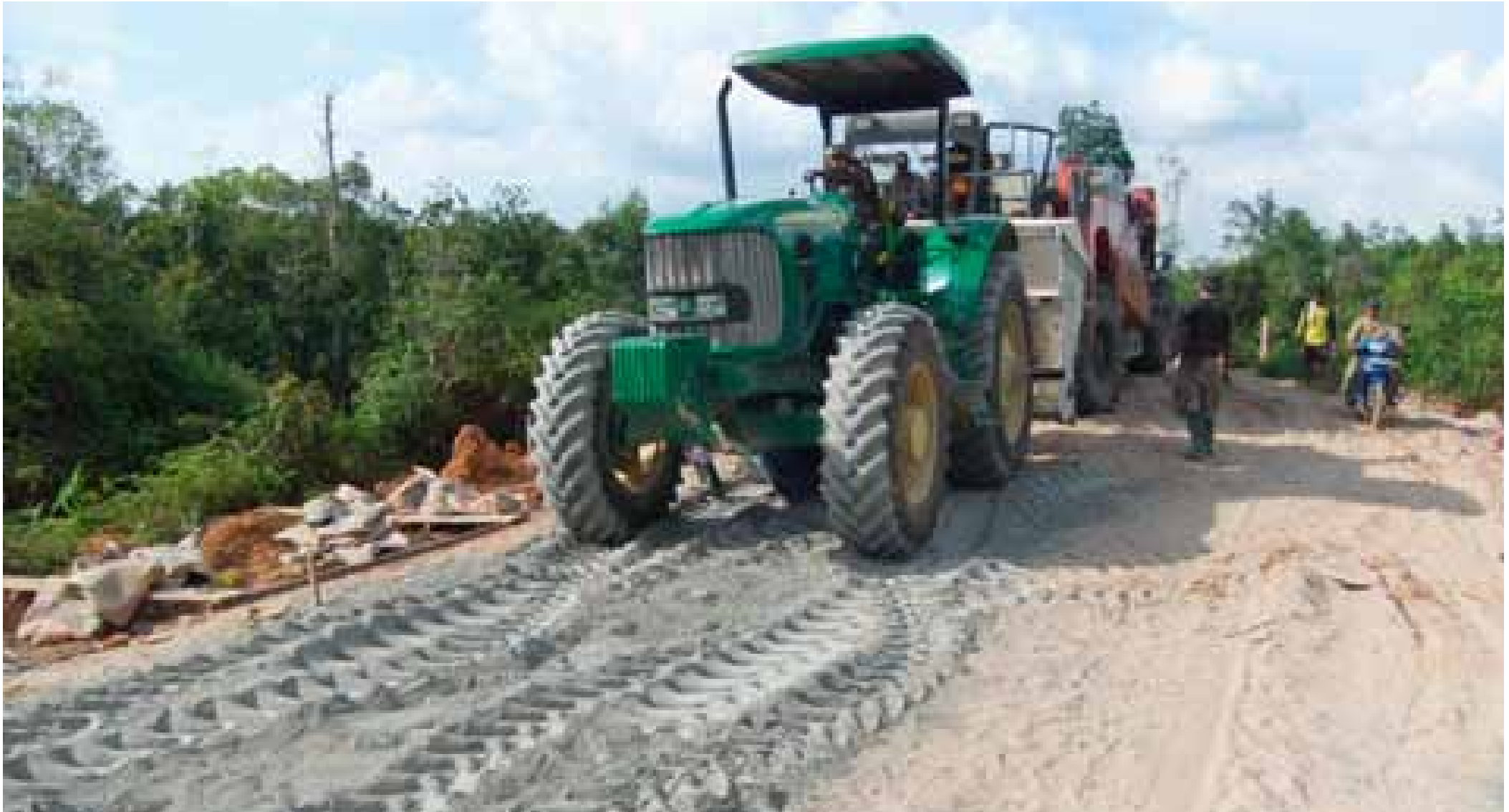
Start of spreading NovoCrete®
