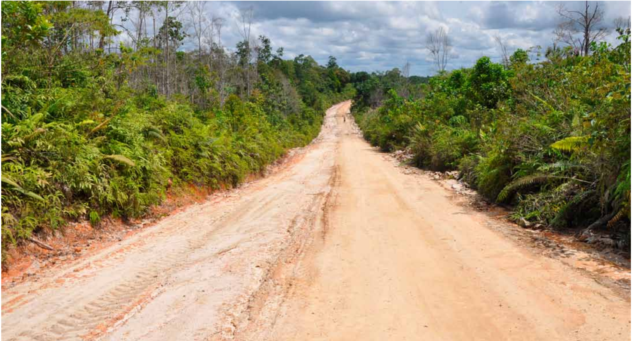
One lane of the finished road
