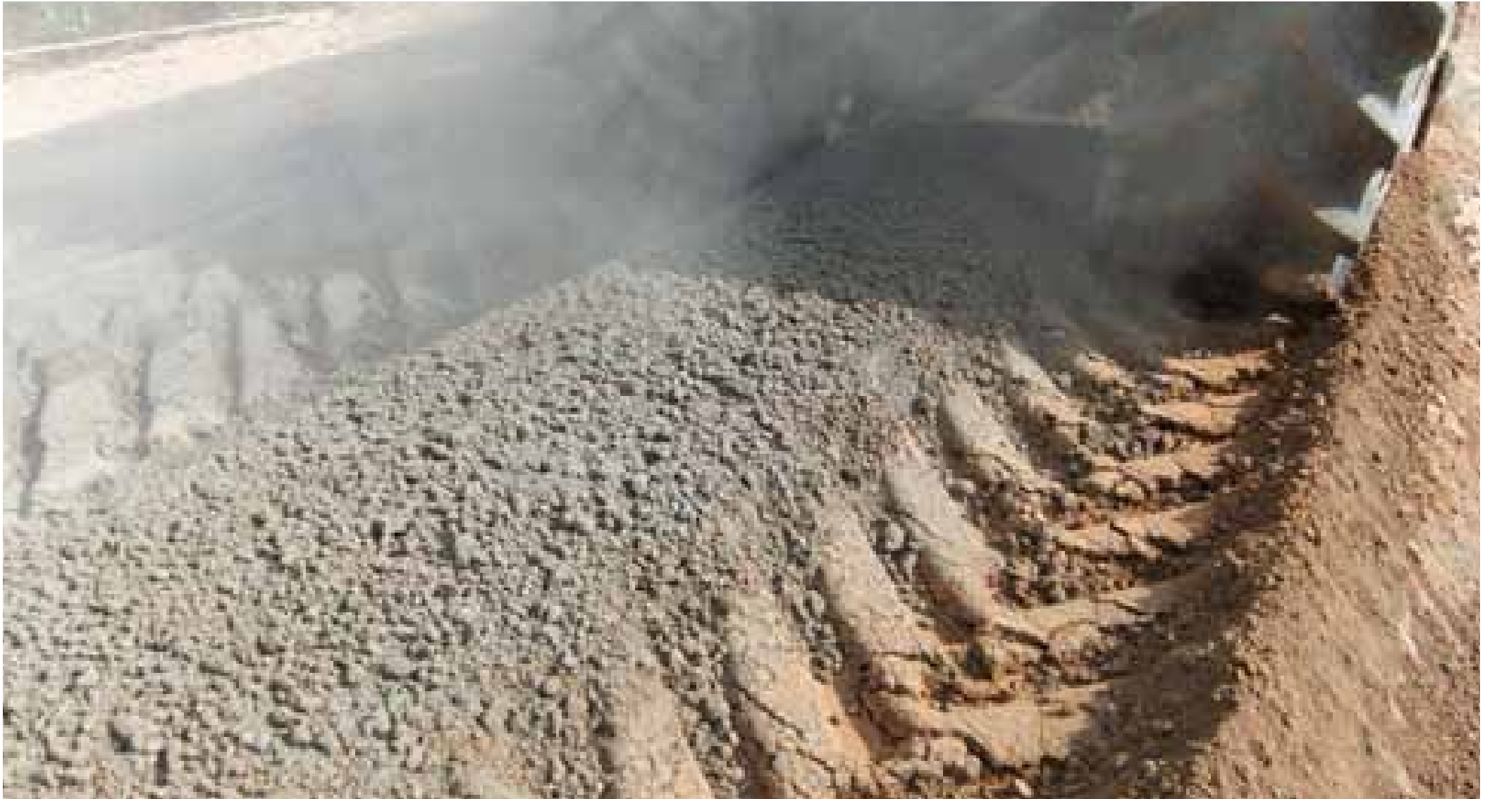
Mixture of soil and binding agent after the first milling procedure
