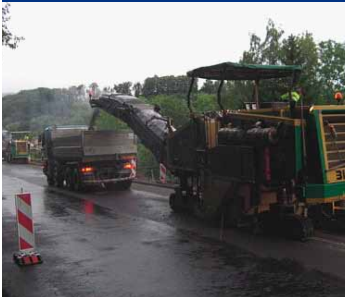
Asphalt milling machine
