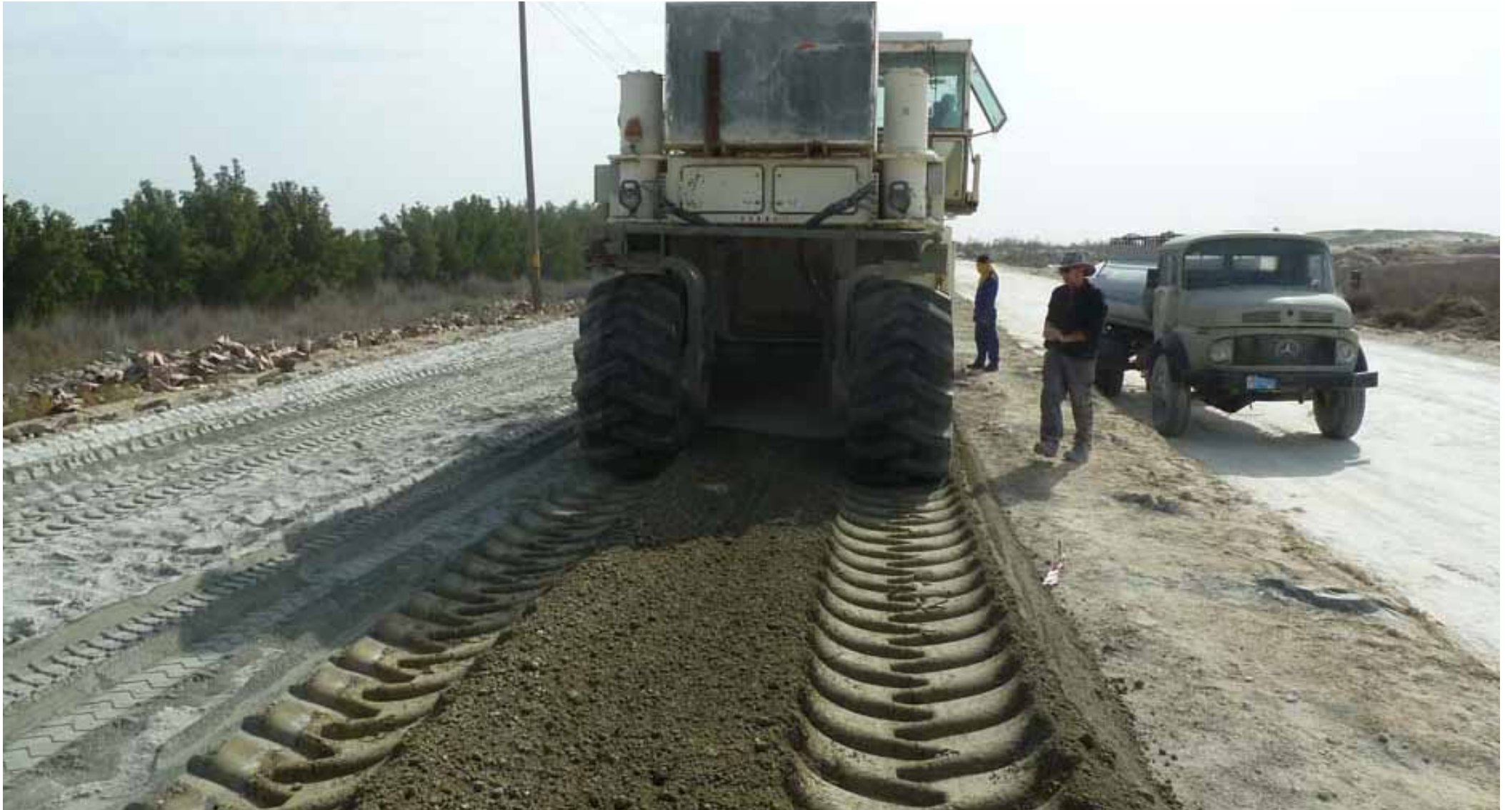
Milling procedure by adding water
