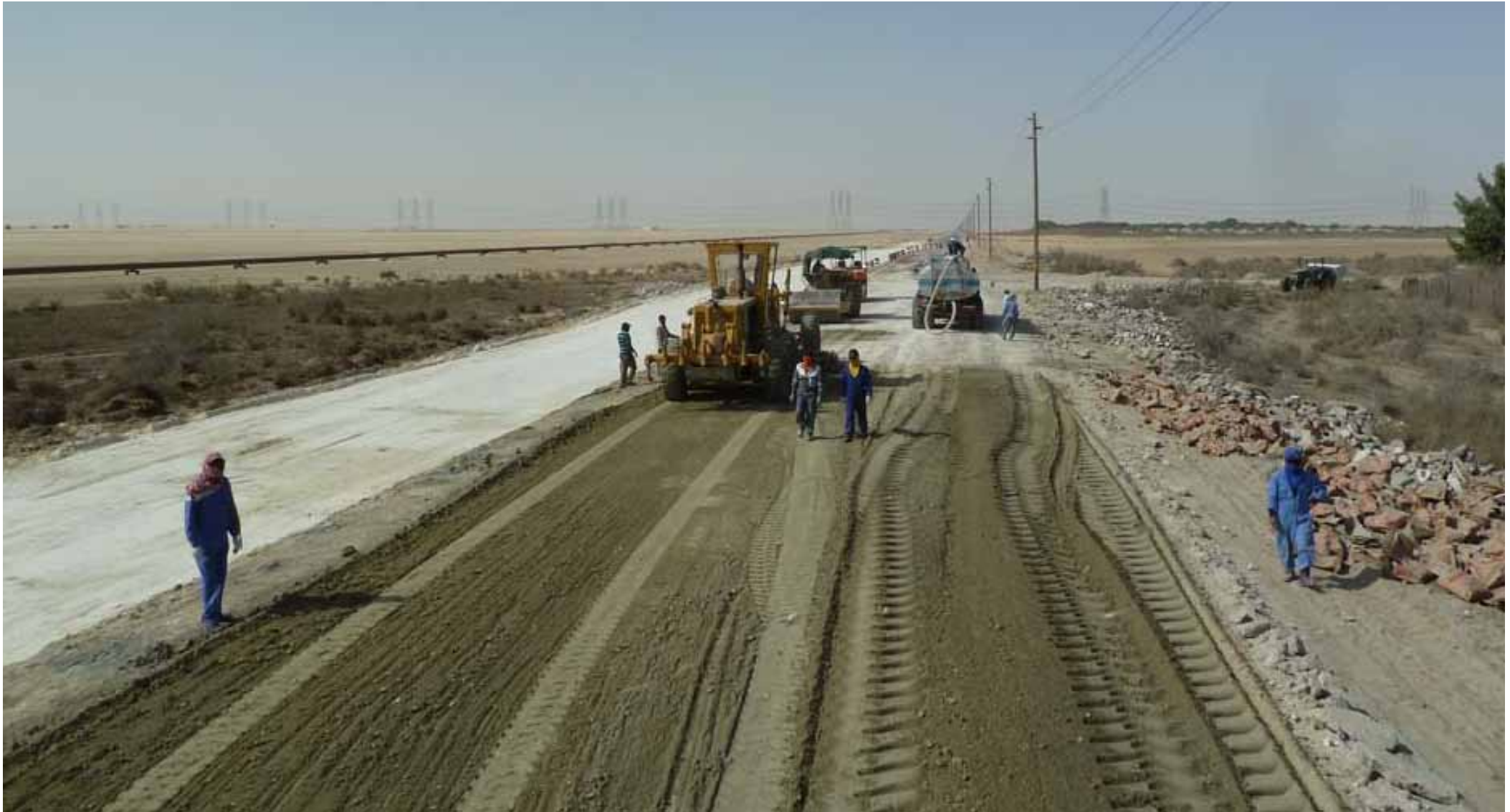
Levelling by using a Grader
