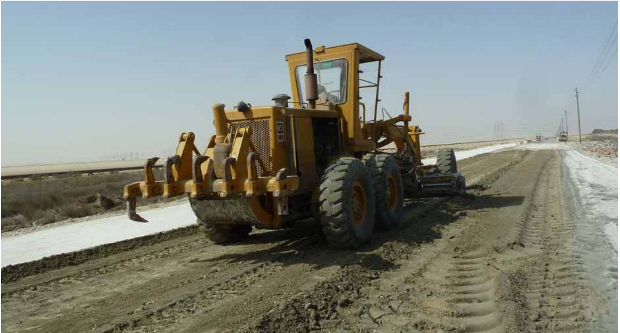
Levelling by using a Grader
