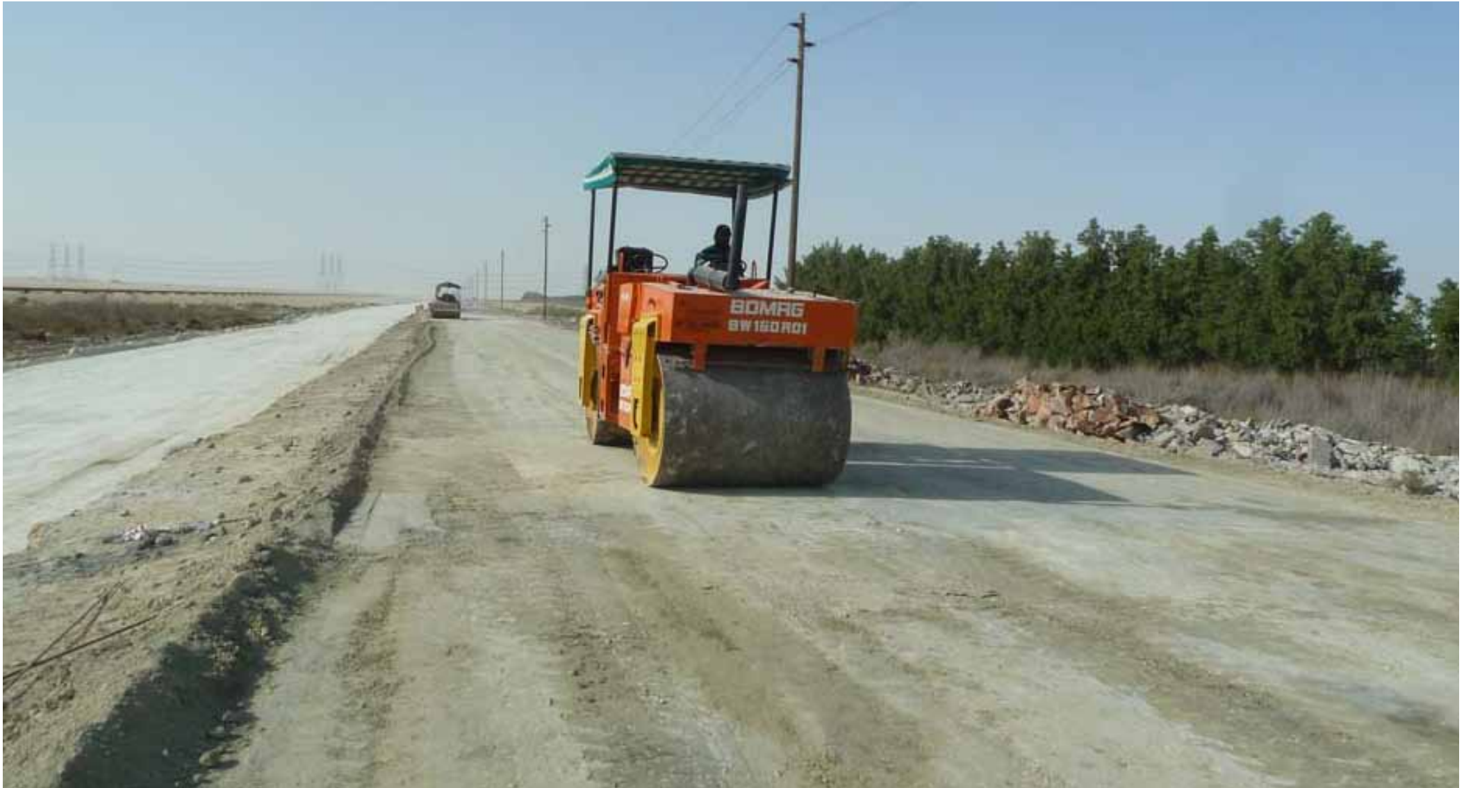
Compaction of the fine level by using a steel drum sollar
