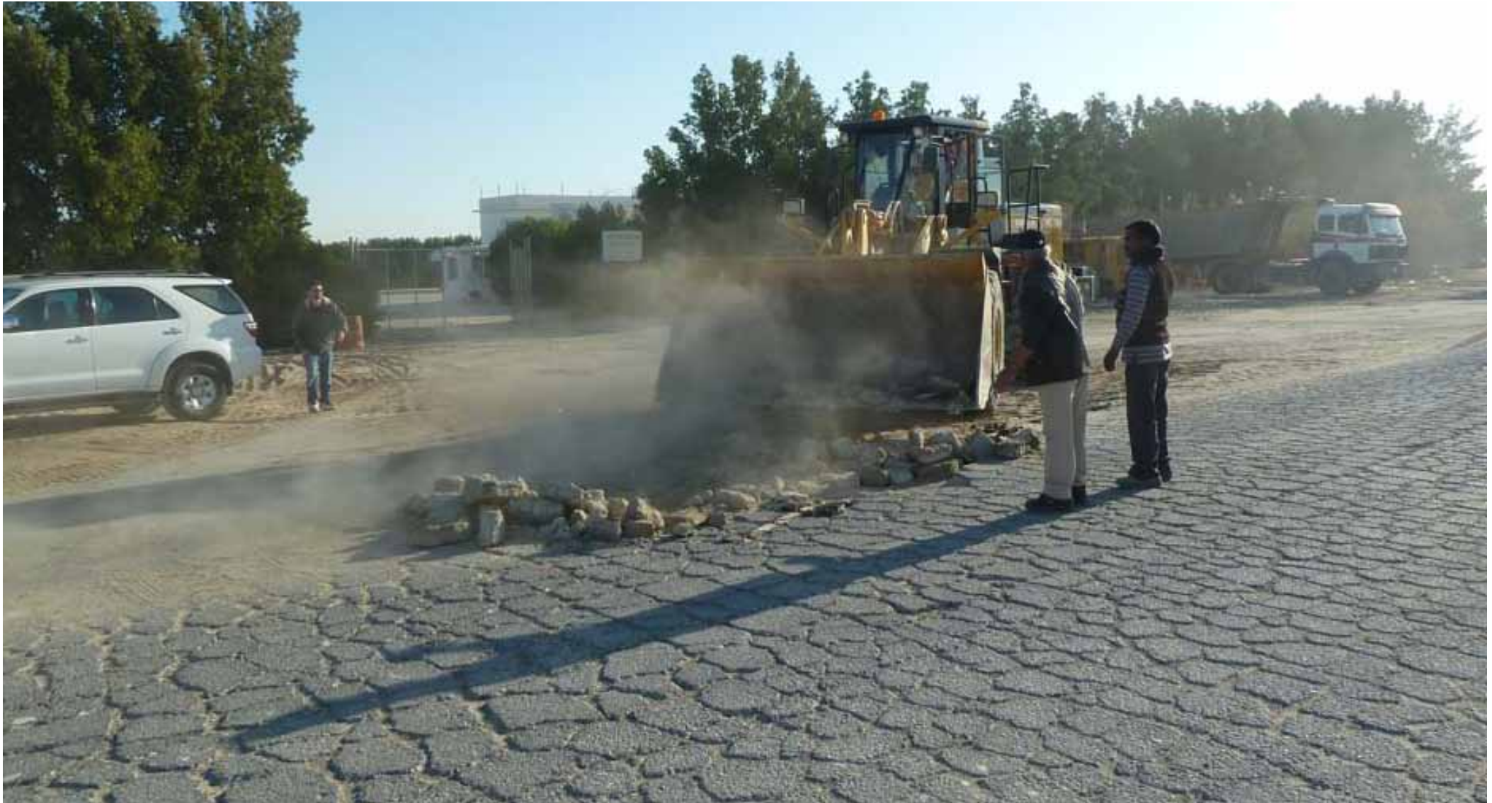
Breaking-up of old asphalt
