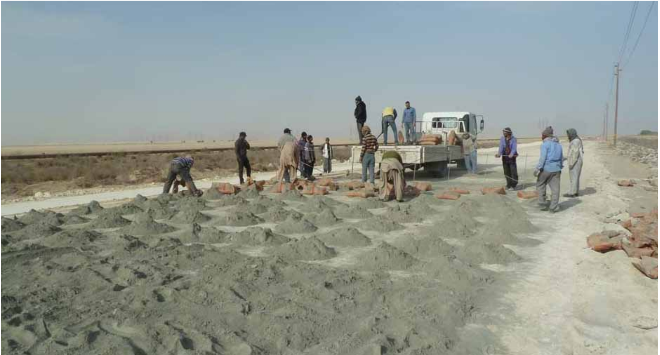
Manually distribution of cement
