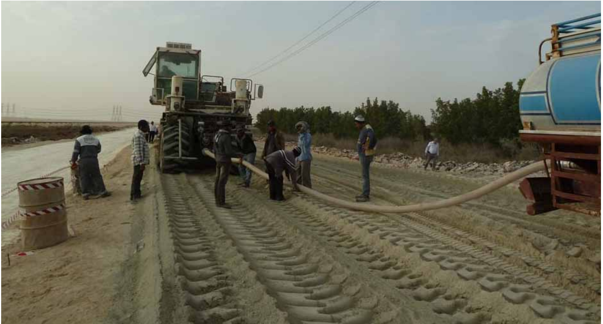
Milling procedure by adding water
