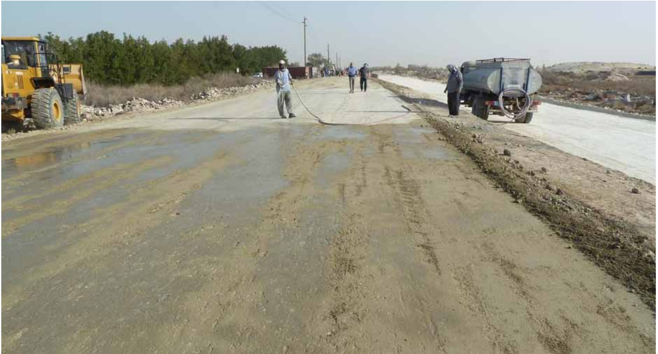
Irrigation of the area
