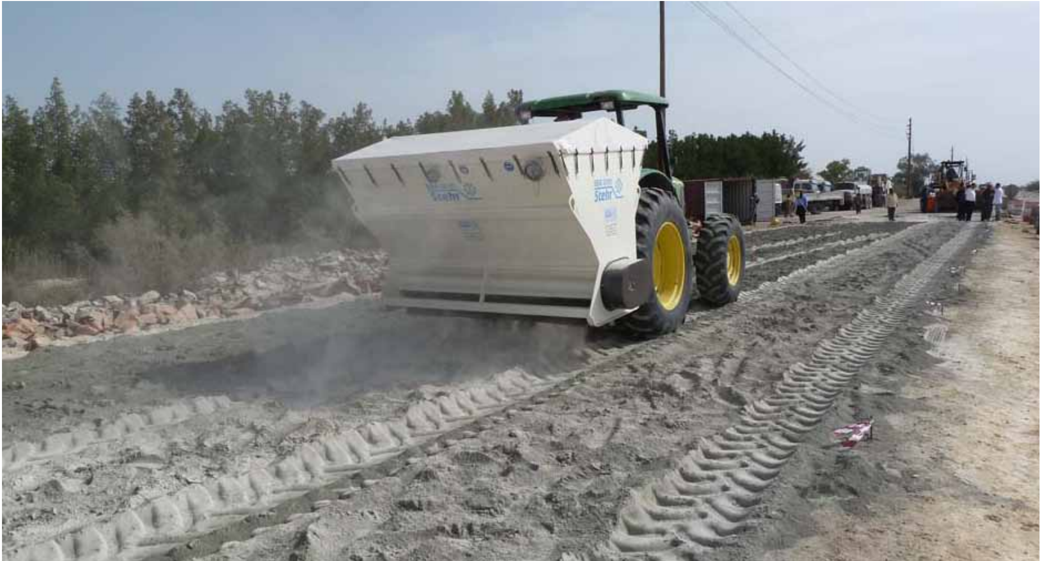
Spreading of NovoCrete
