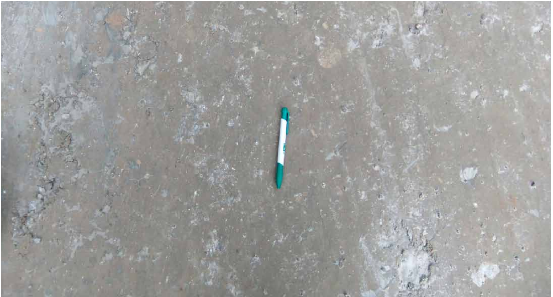
Surface of finished area
