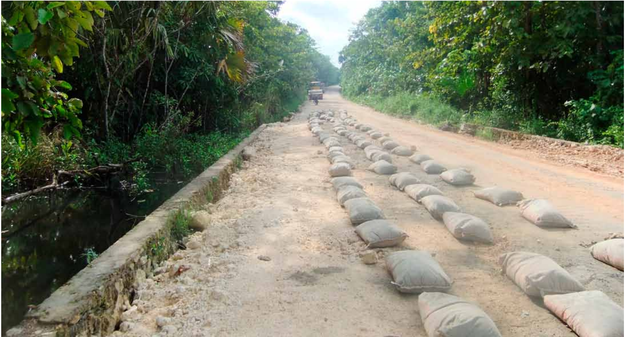
Distribution of cement bags
