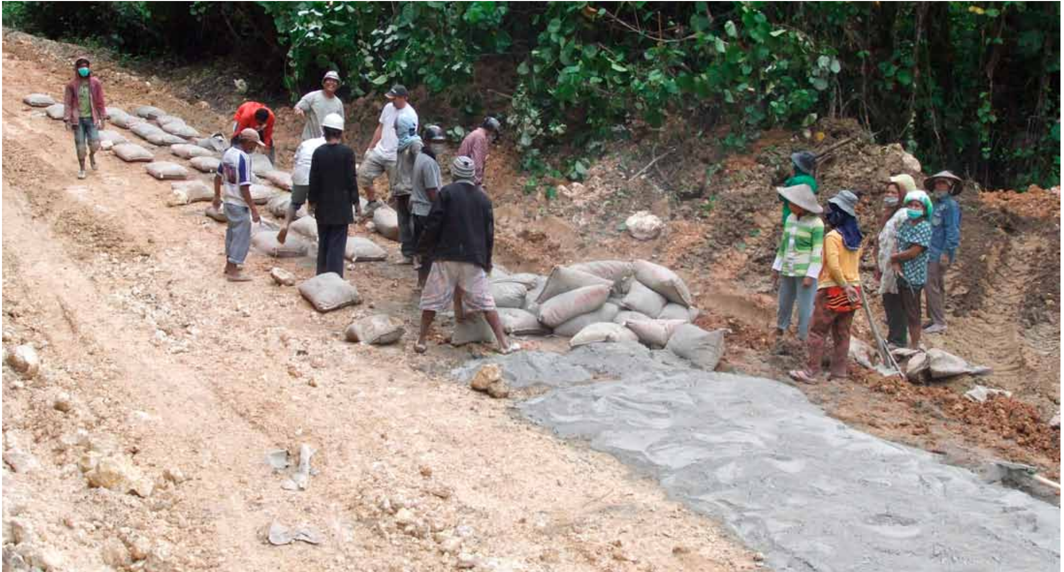
Distribution of cement bags
