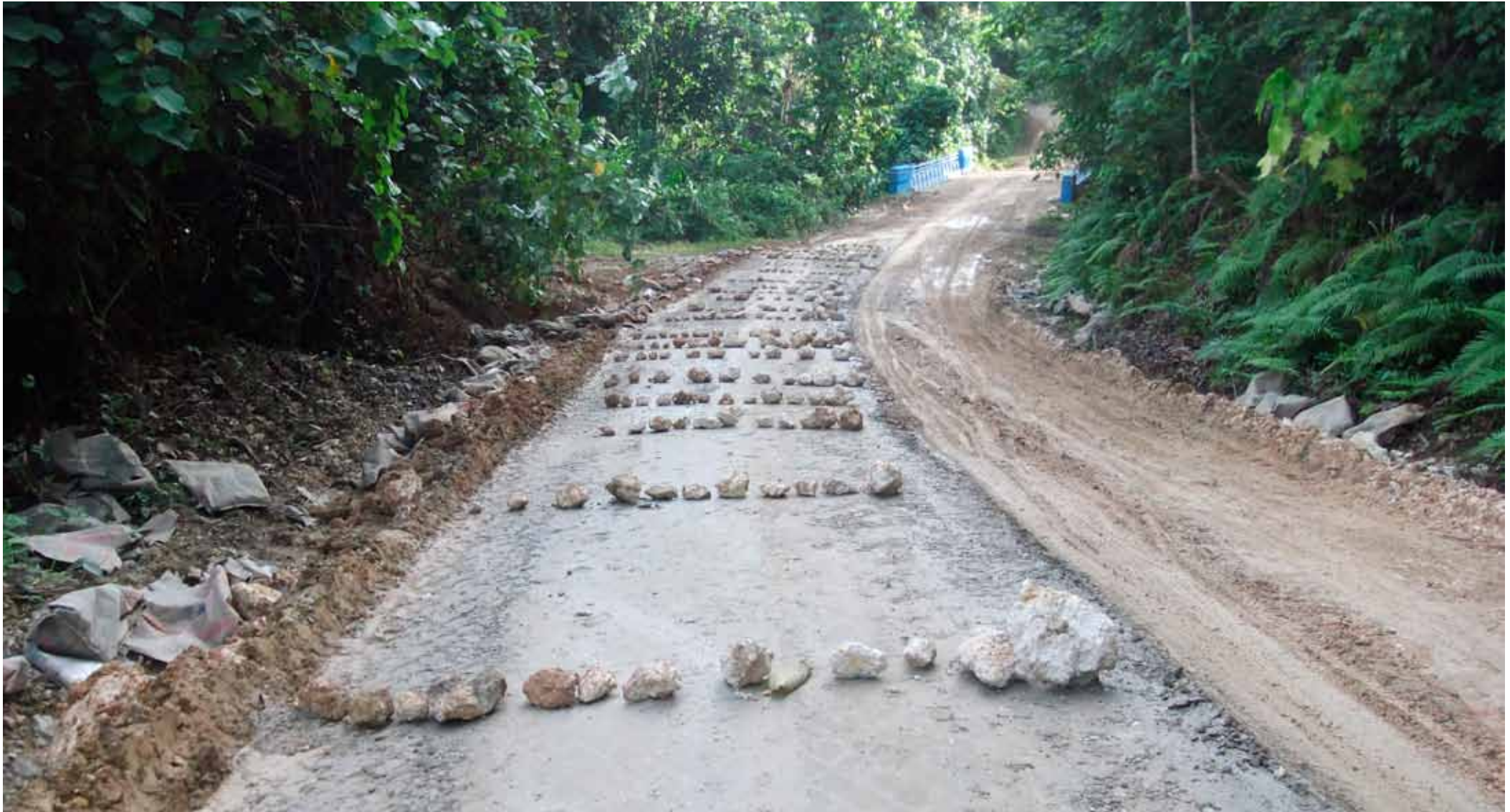
Finished area blocked for traffic
