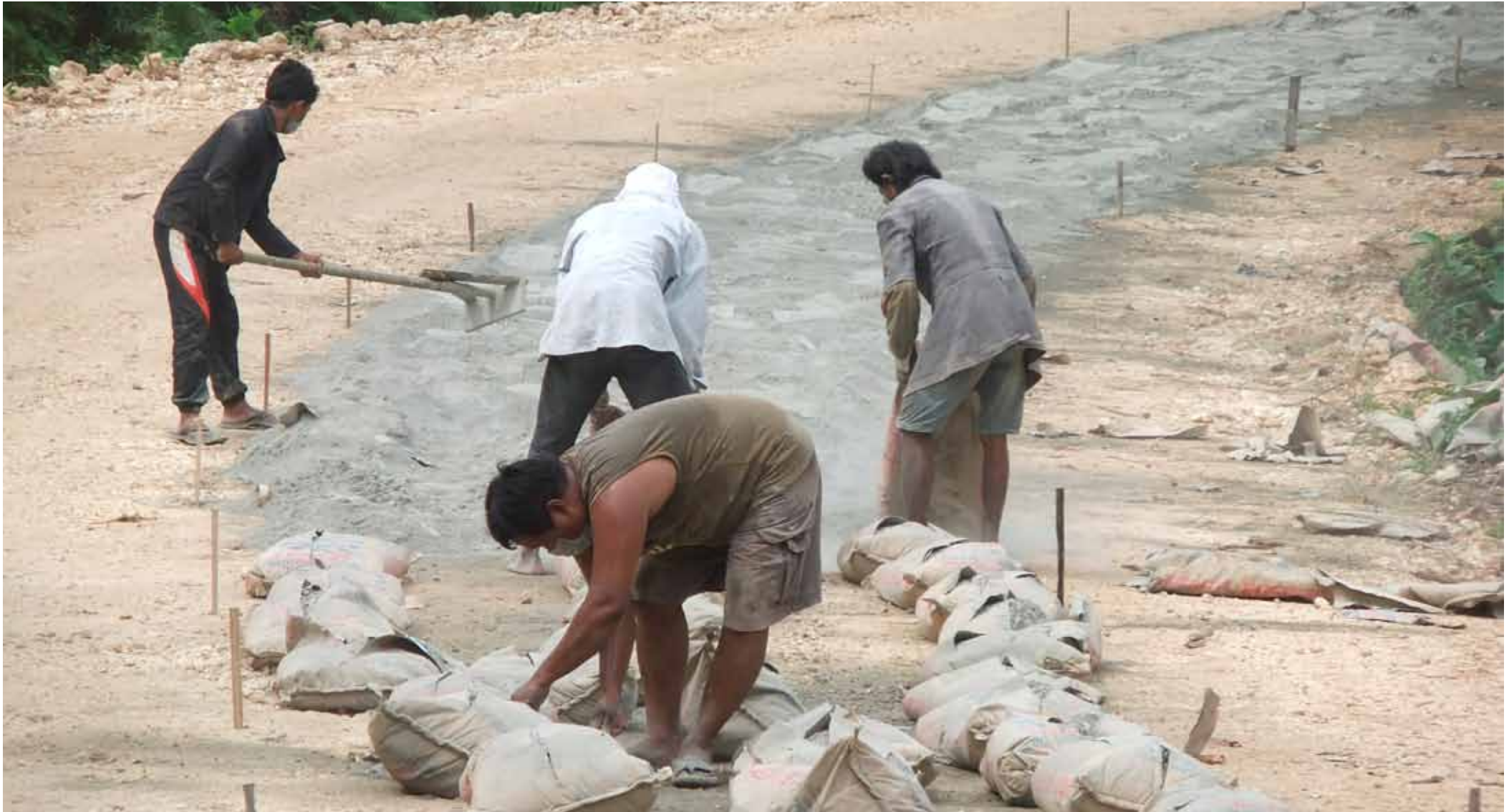
Manually distribution of cement
