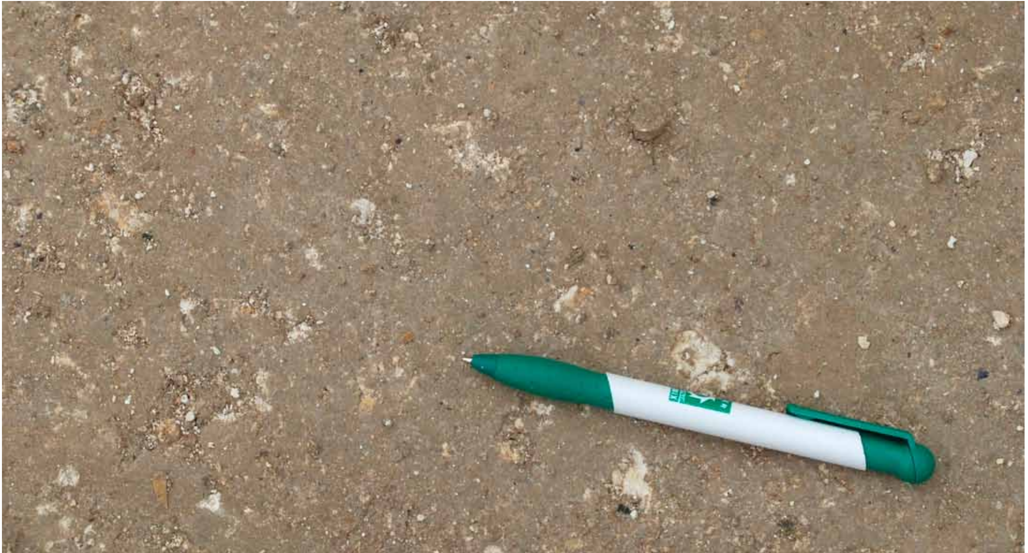
Surface of finished area
