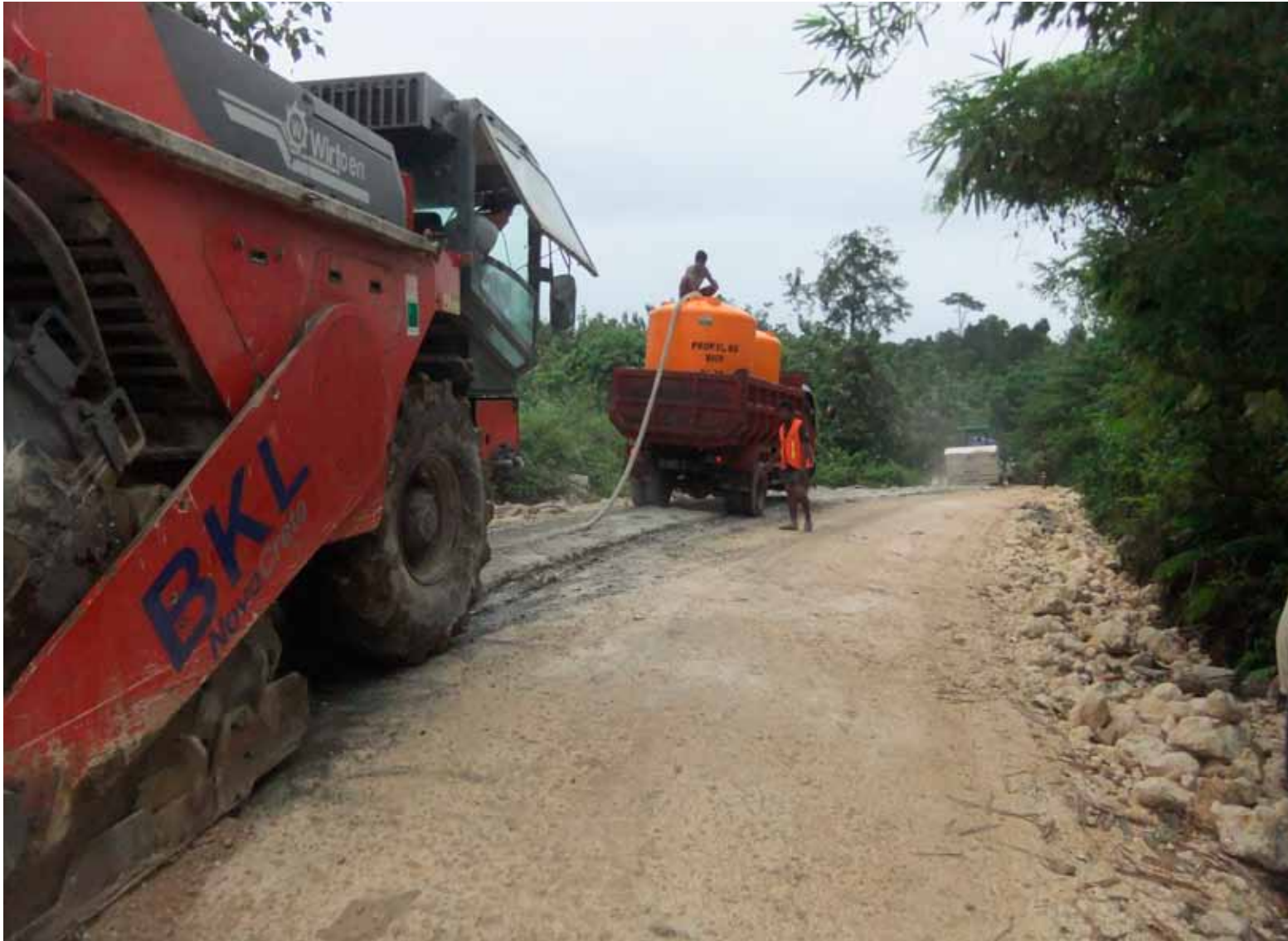
Milling procedure
