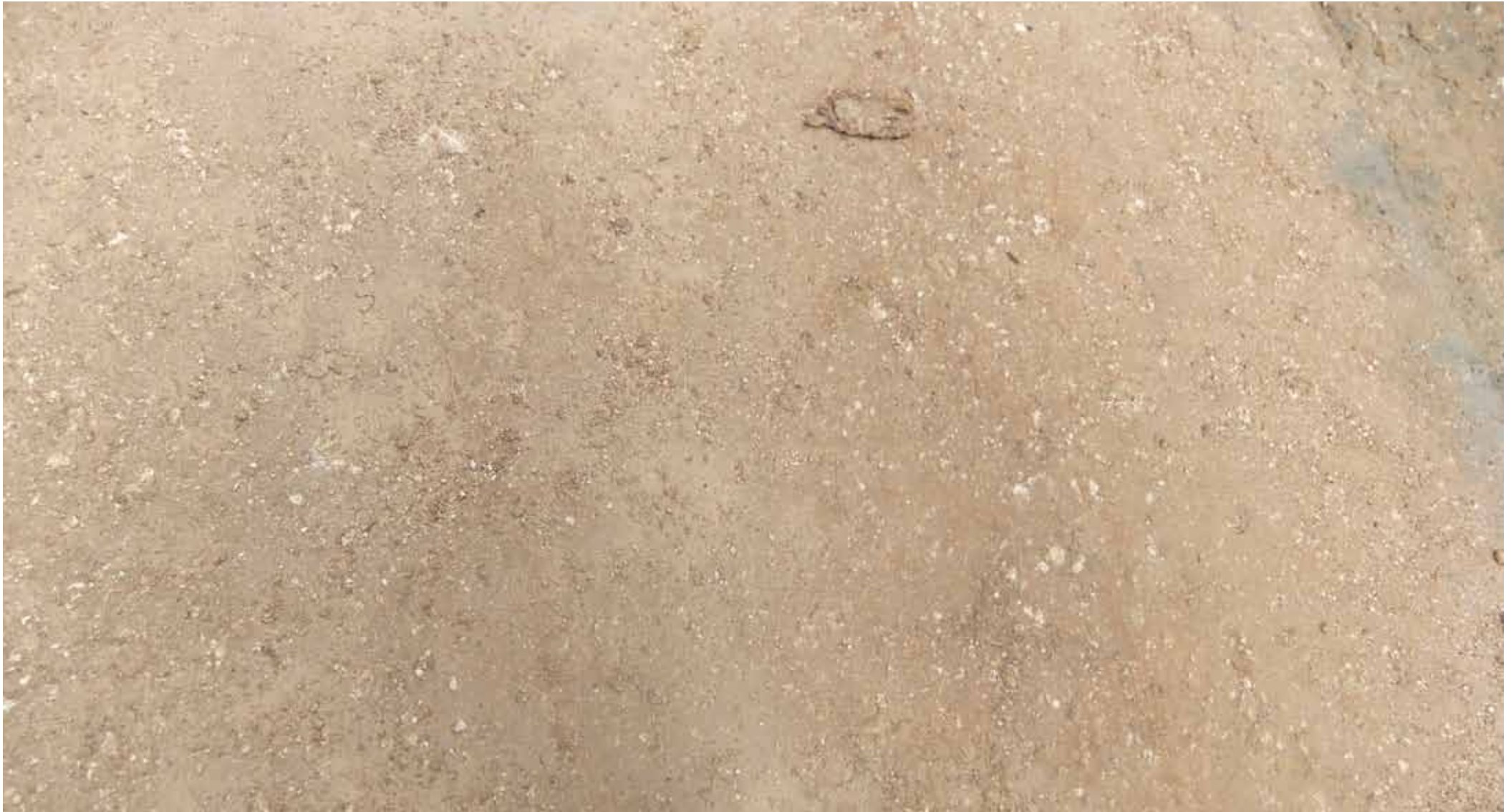
Close-up of the finished surface
