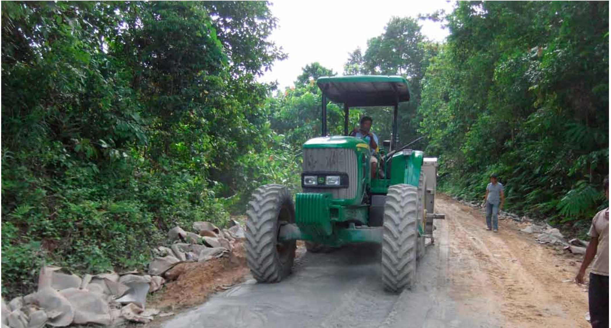
Spreading of NovoCrete
