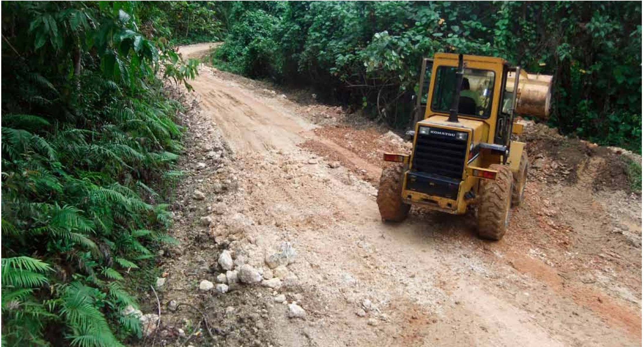
Preparation of the rough level
