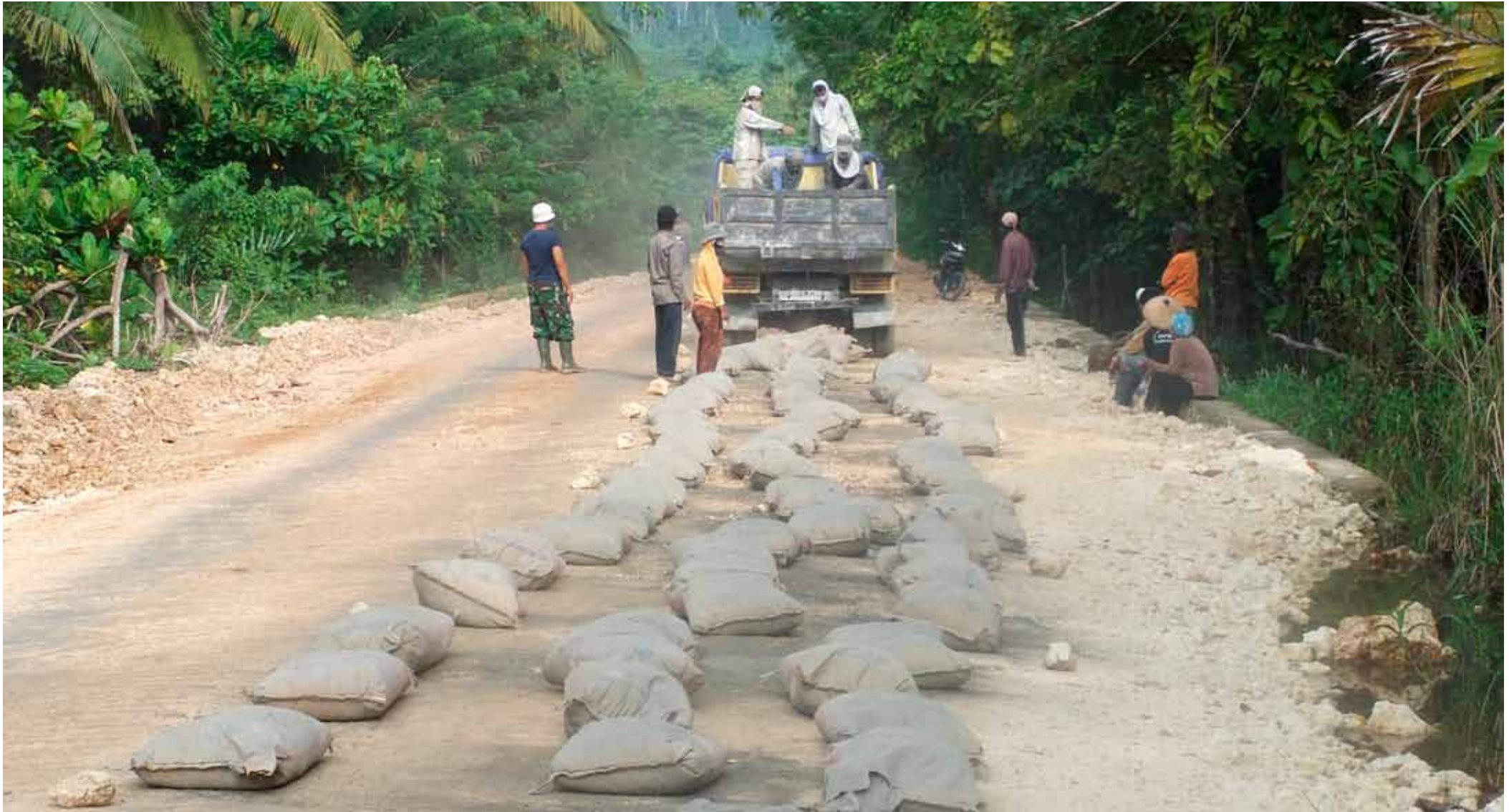
Distribution of cement bags
