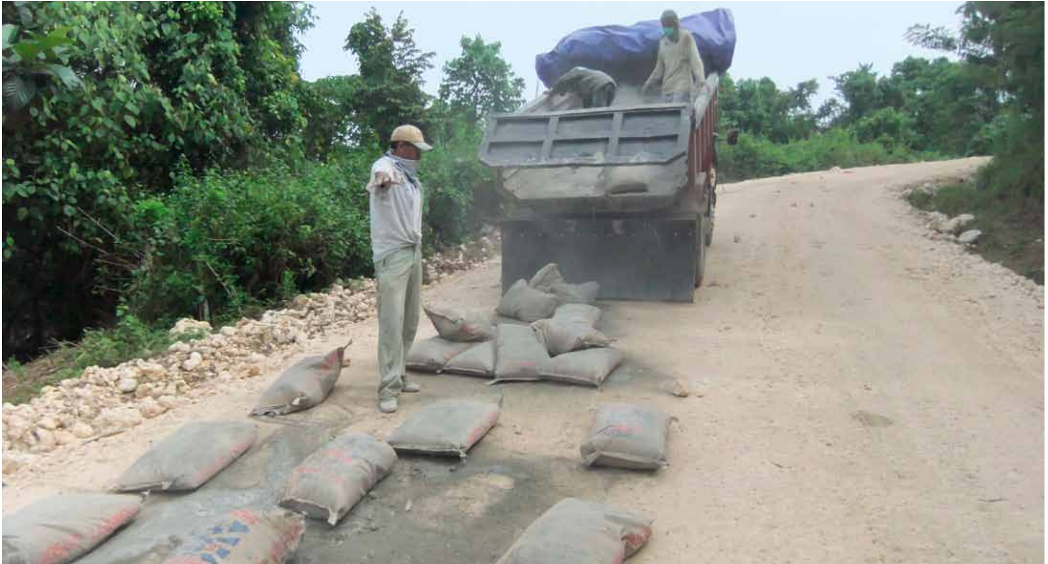
Distribution of cement bags
