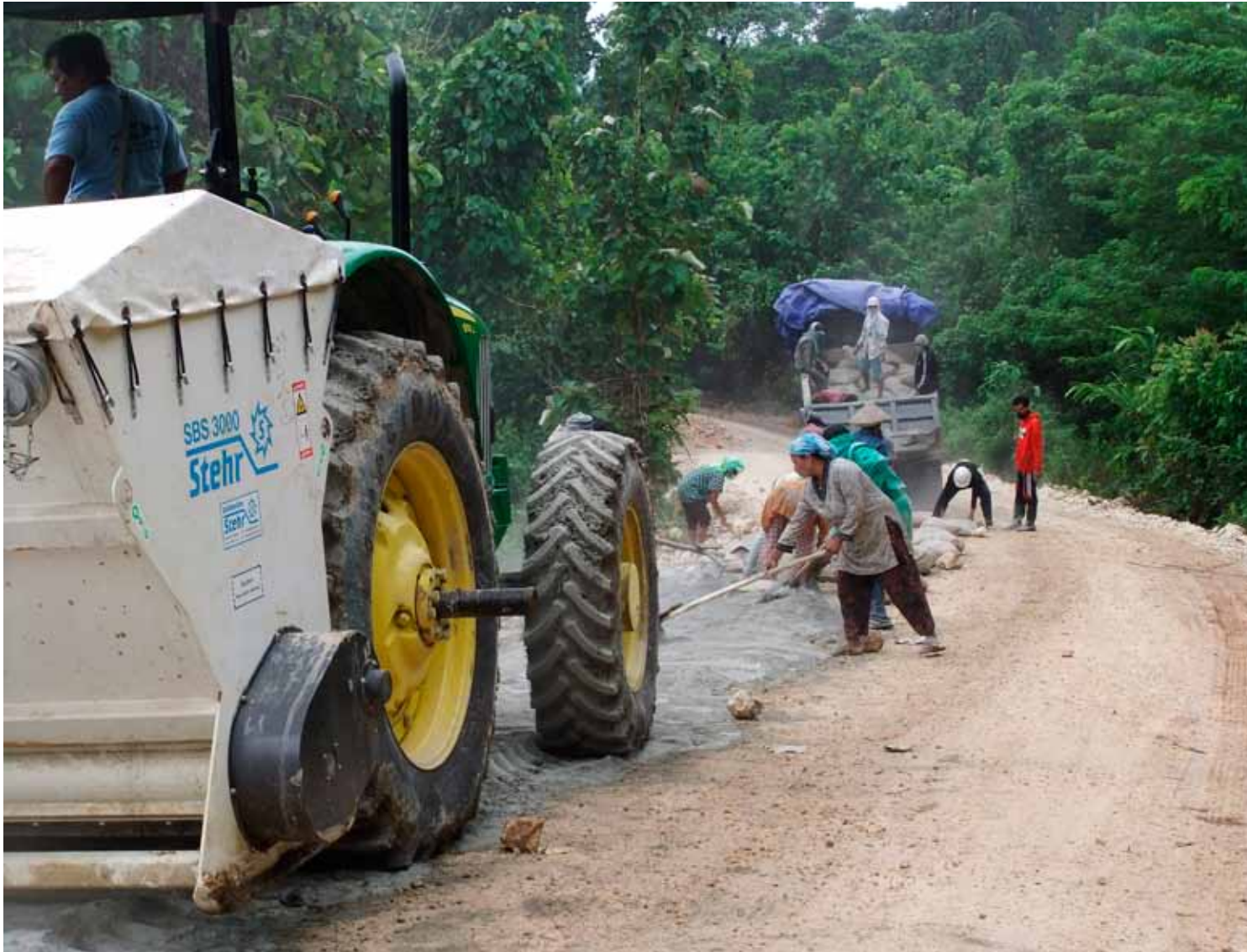
Spreading of NovoCrete
