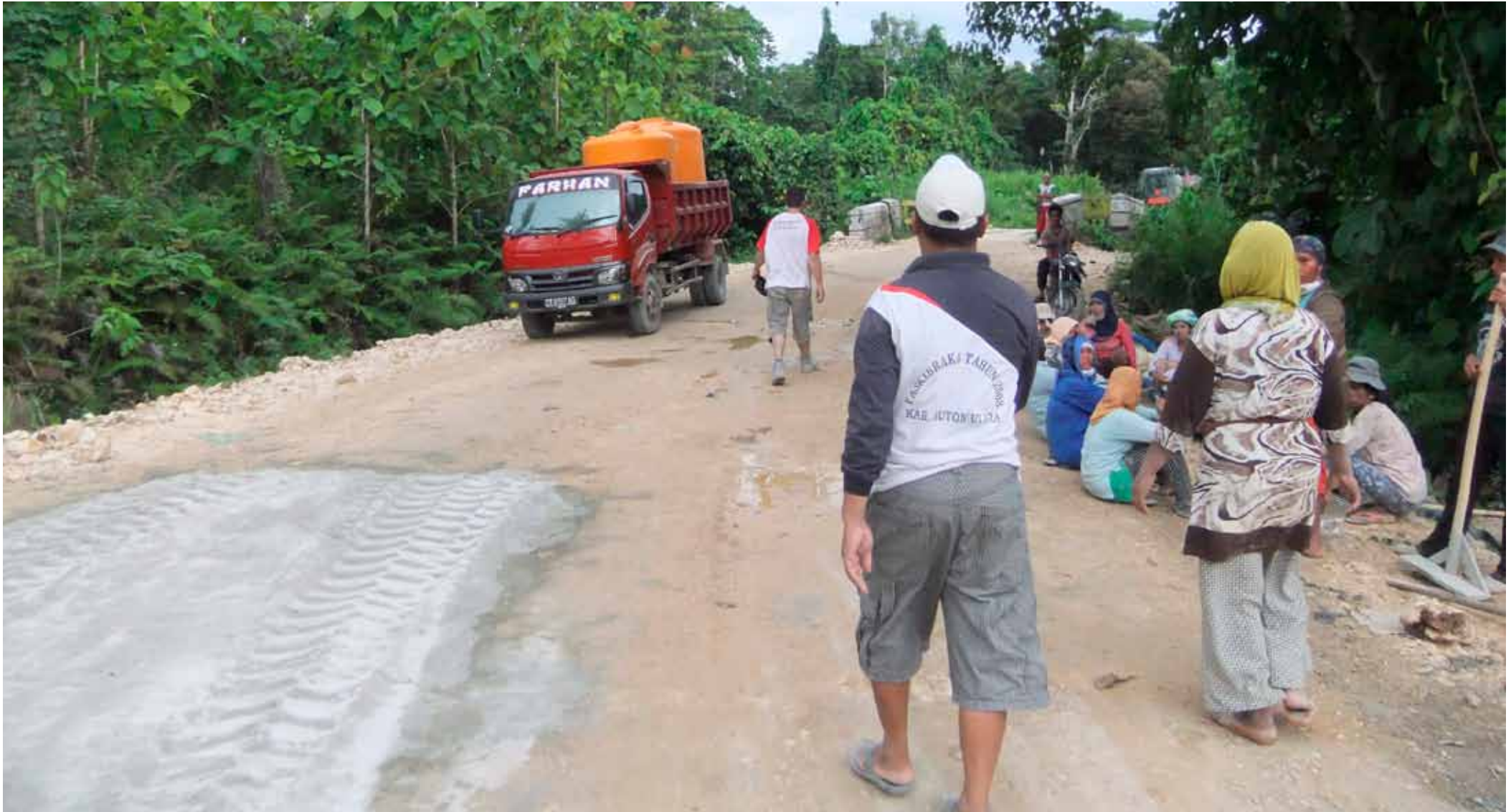
Spreading of cement
