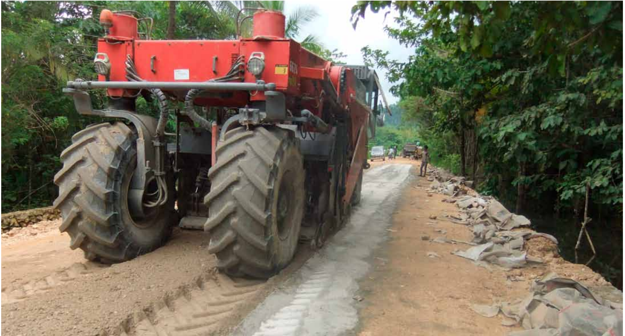
Milling procedure
