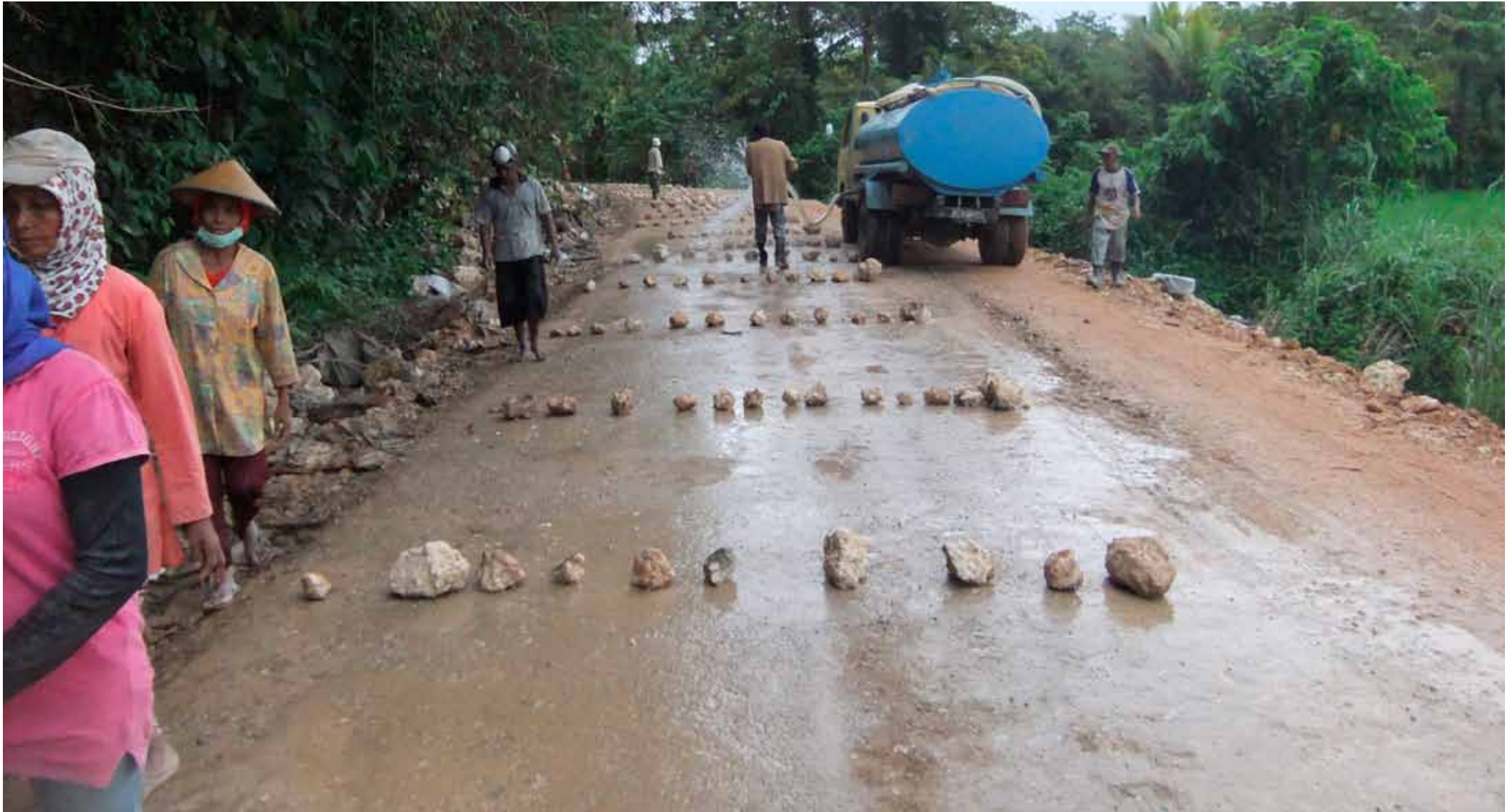
Finished area blocked for traffic
