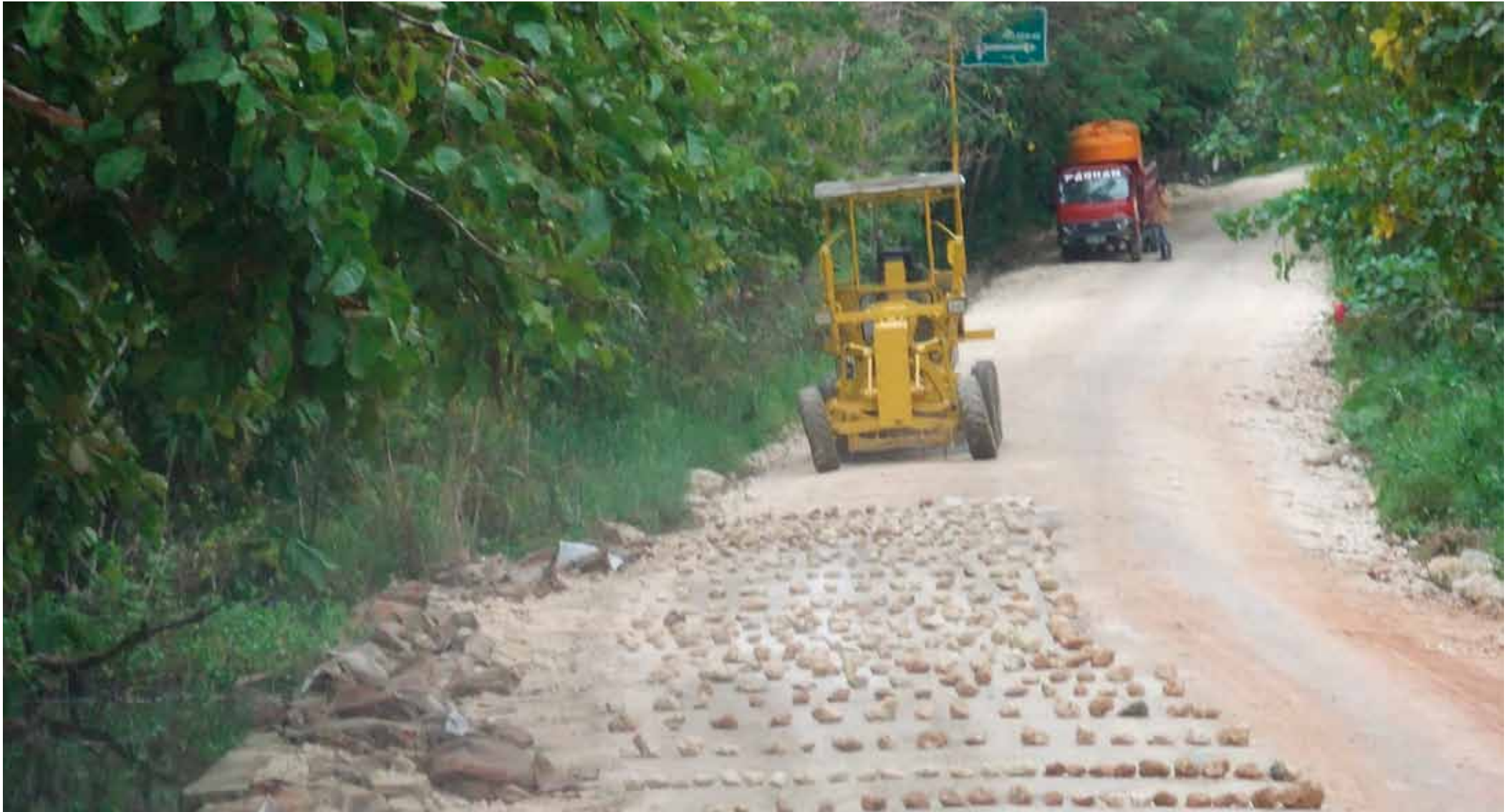
Finished area blocked for traffic
