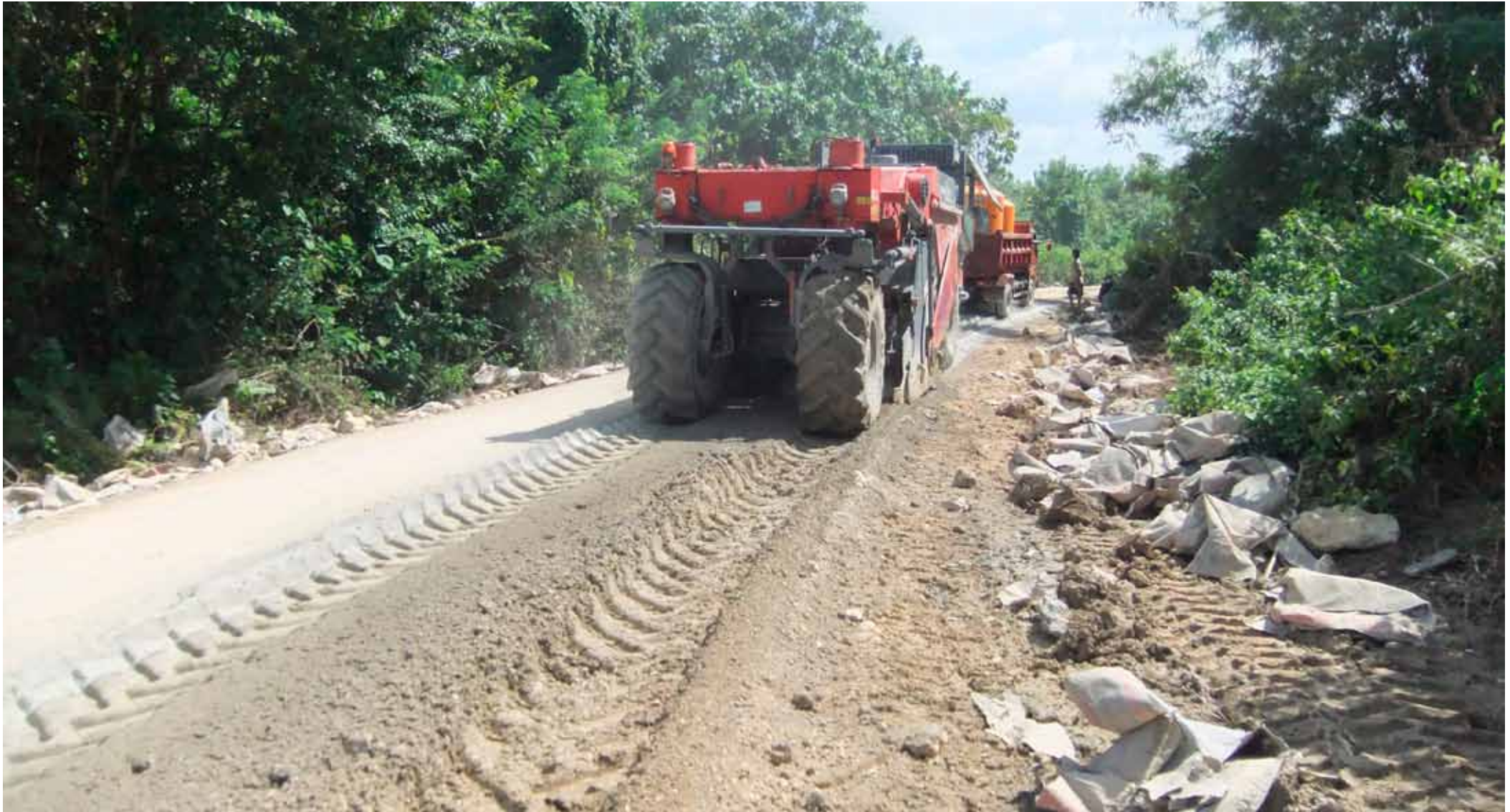
Milling procedure
