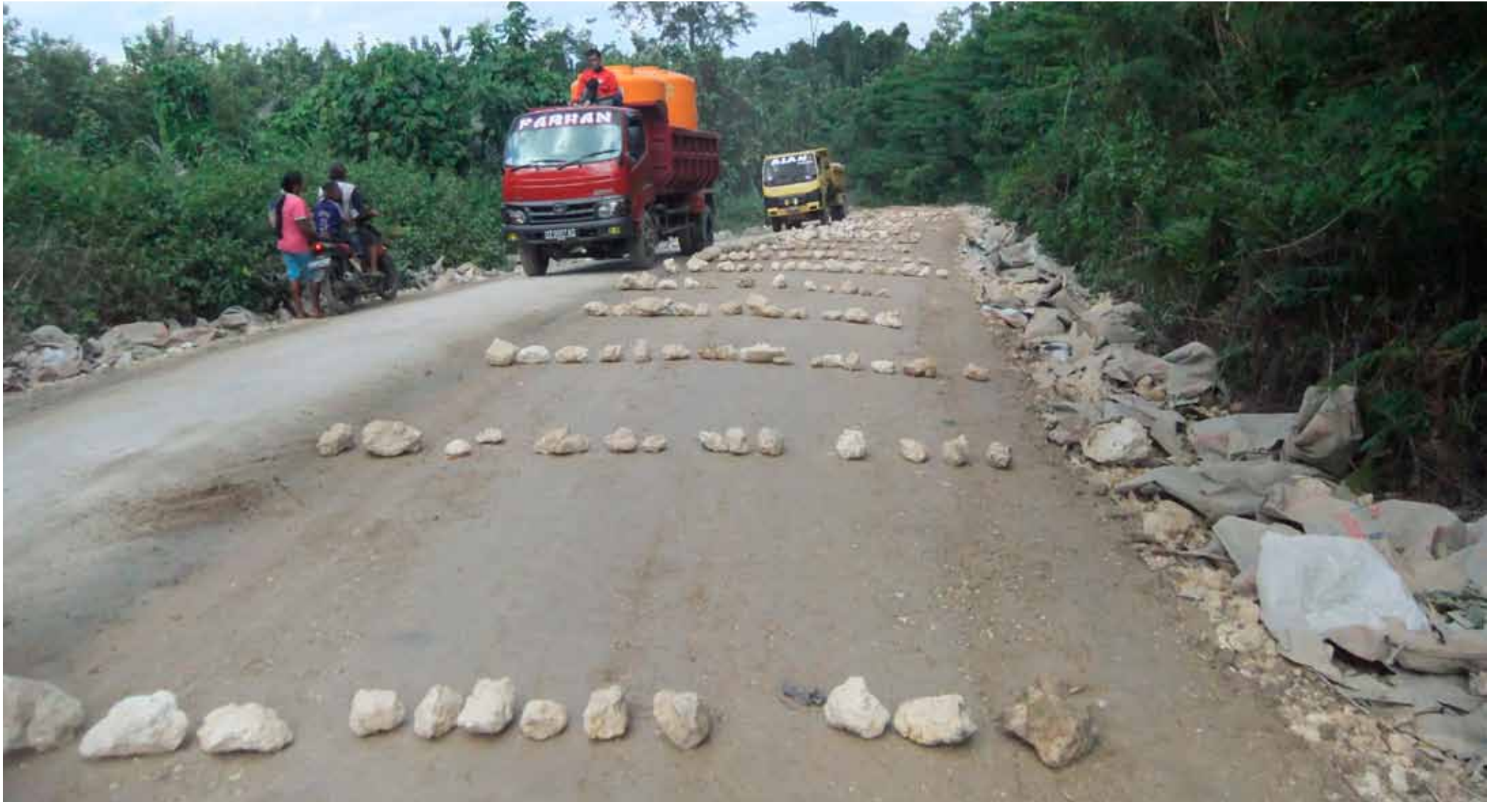
Finished area blocked for traffic
