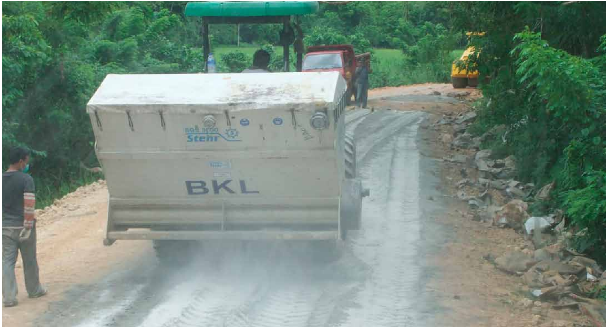
Spreading of NovoCrete
