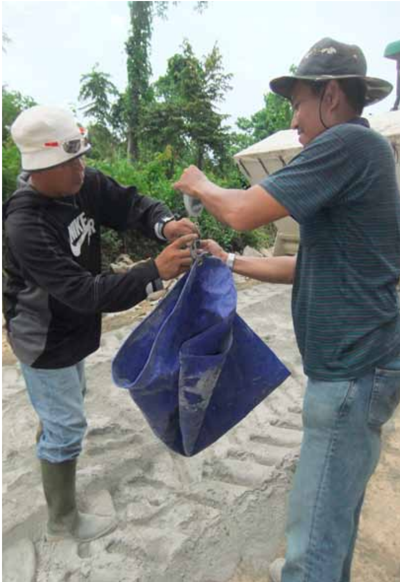
Check of spreaded amount of NovoCrete
