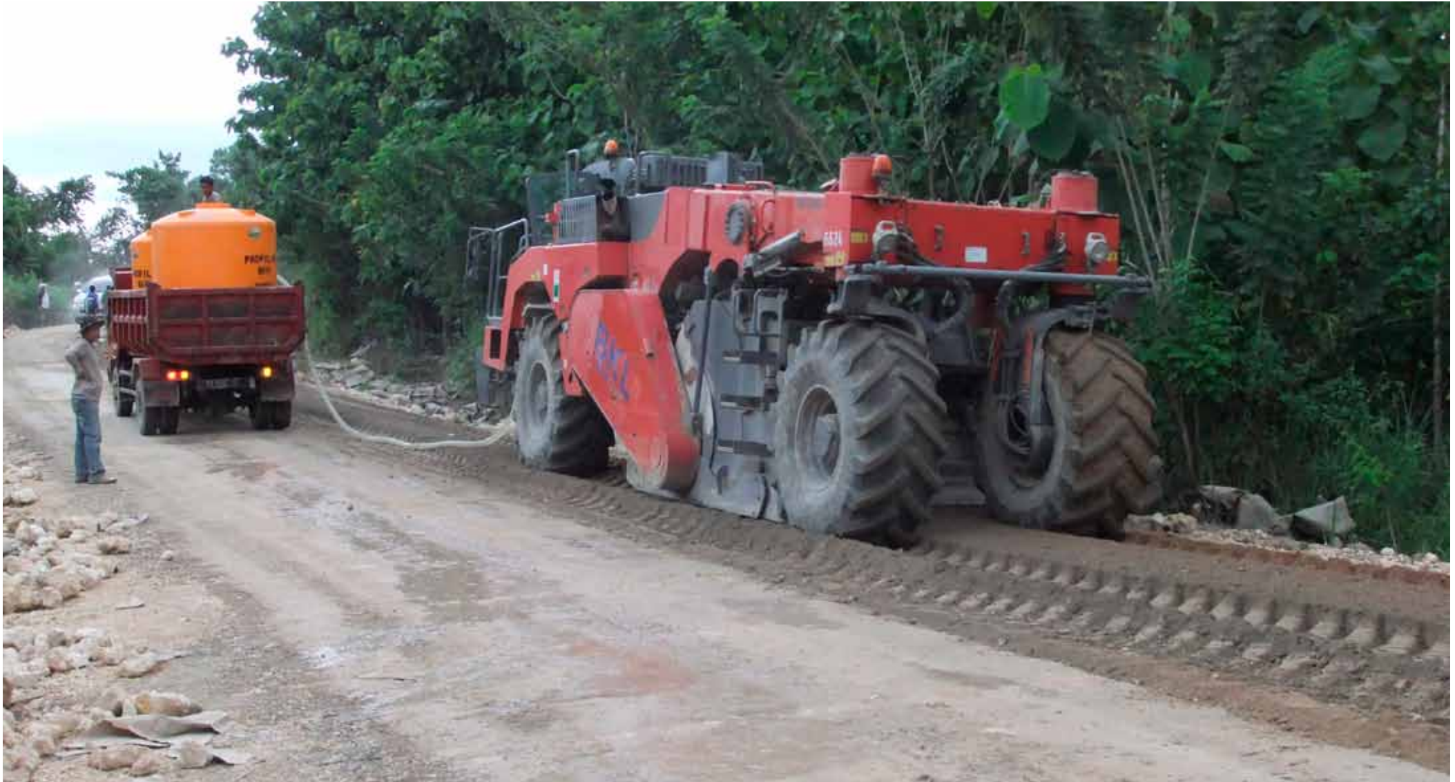
Milling procedure
