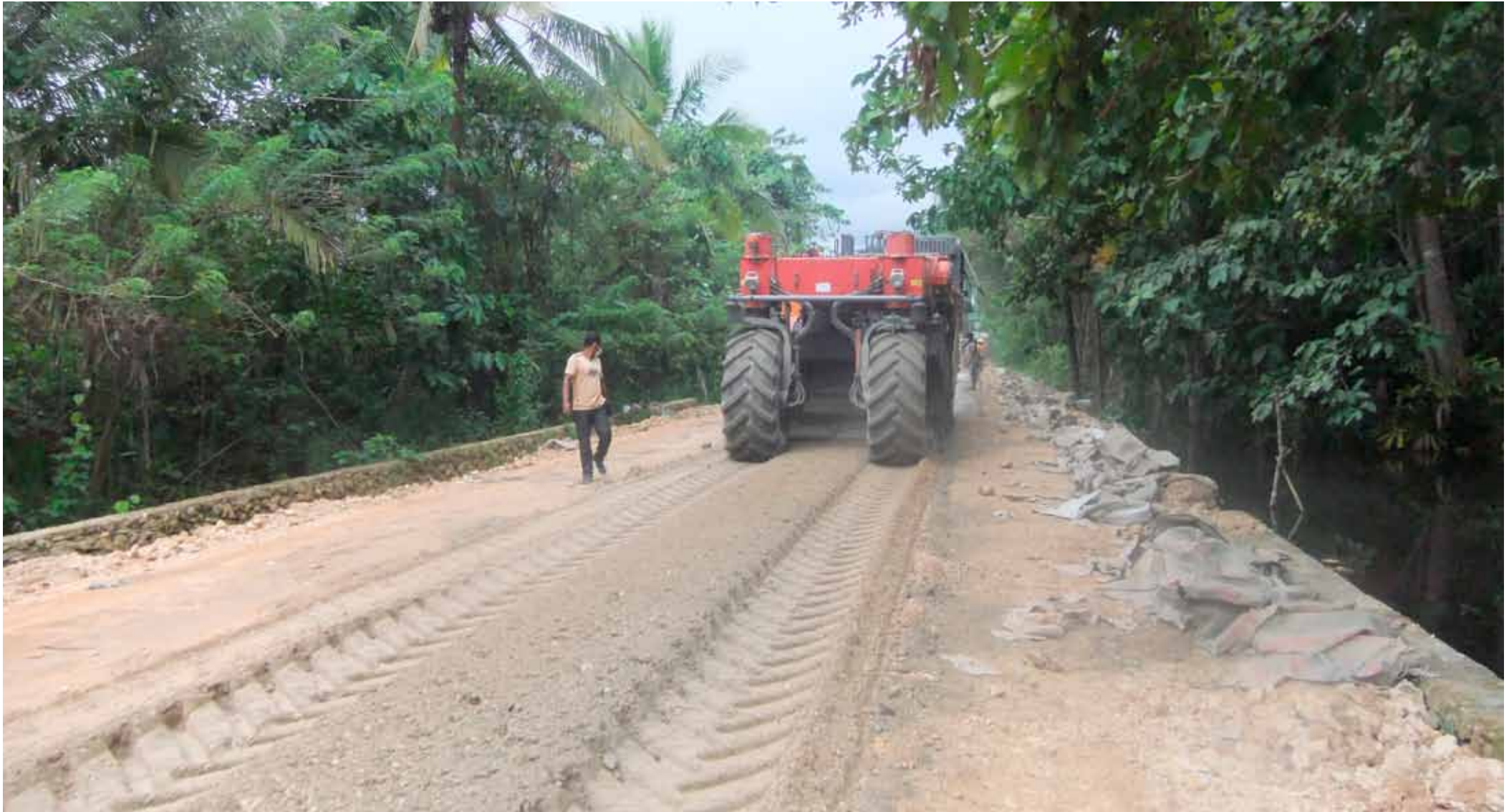
Milling procedure
