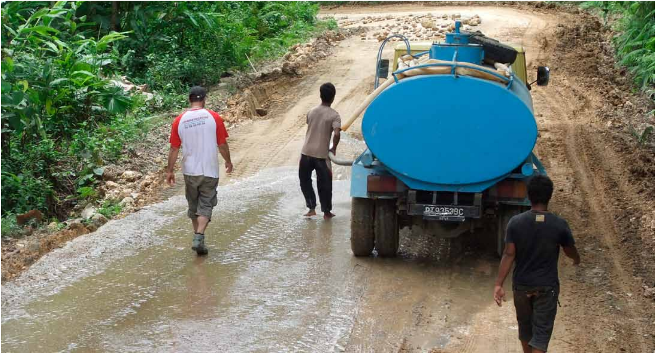
Irrigation of the surface
