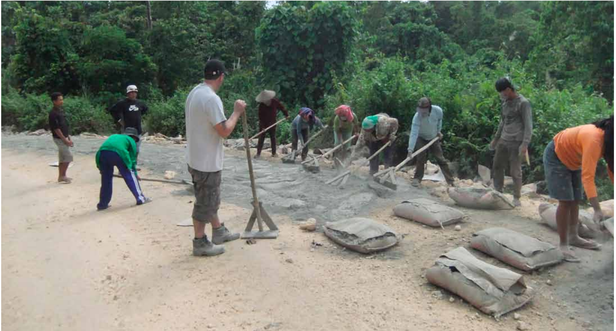
Manually distribution of cement
