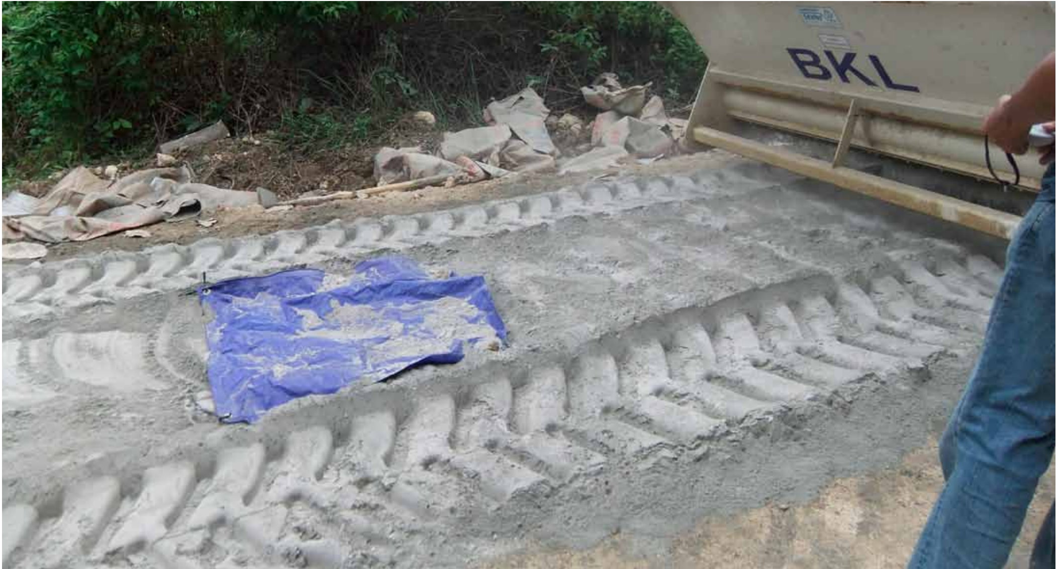
Check of spreaded amount of NovoCrete
