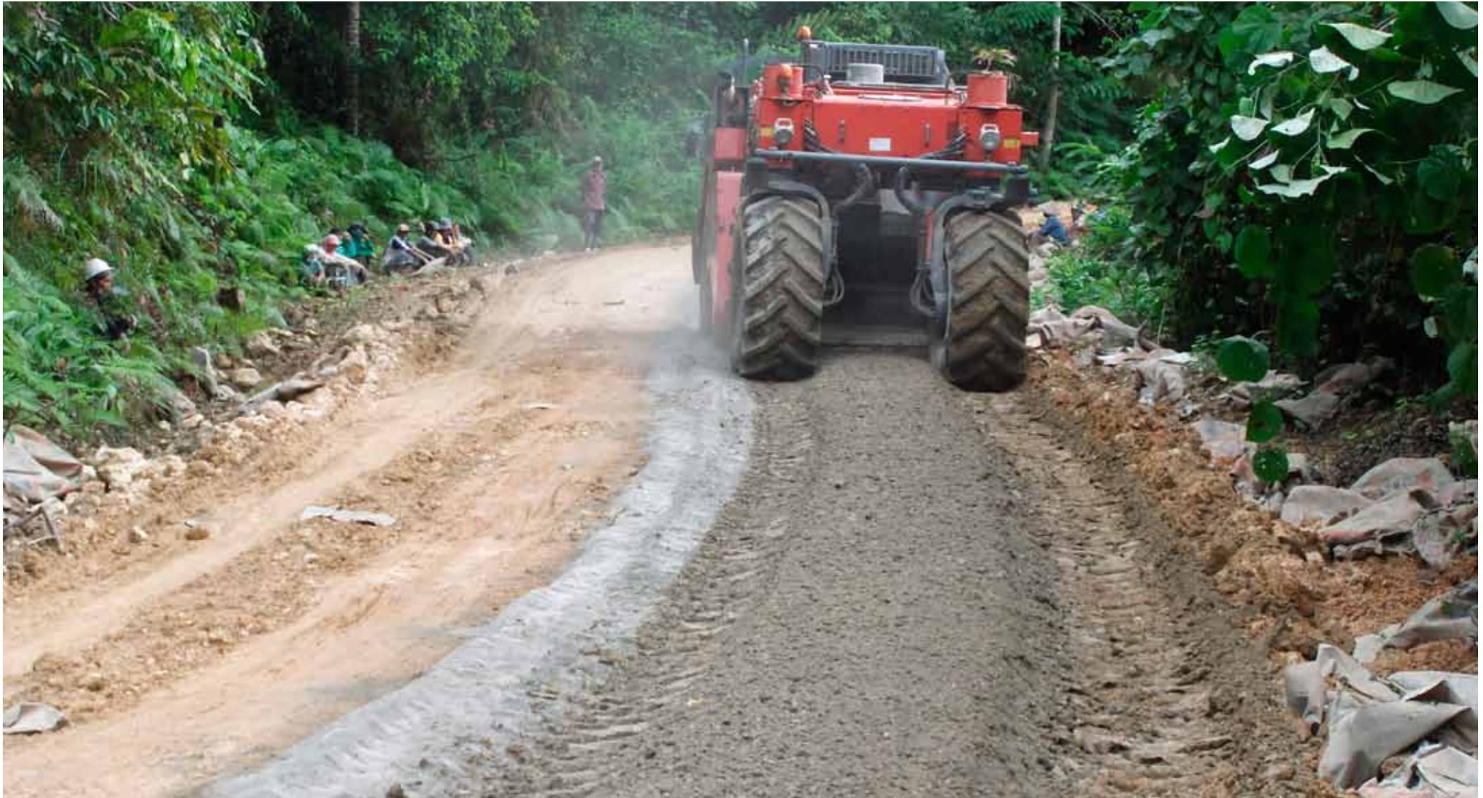
Milling procedure
