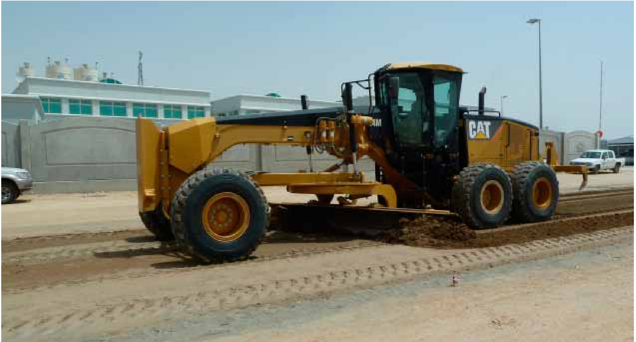
Levelling with a Grader
