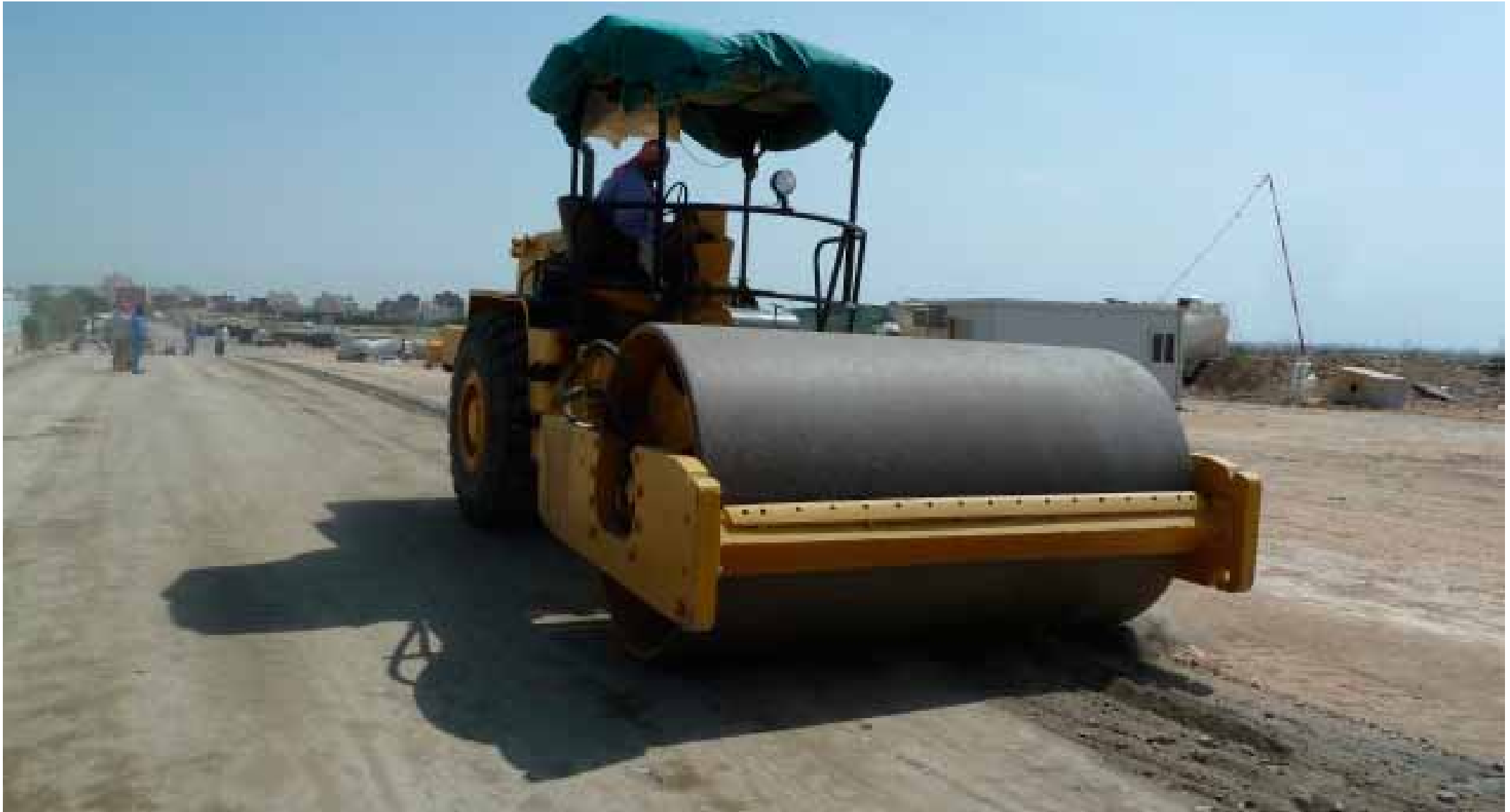
Dynamic and static compaction with a steel drum roller
