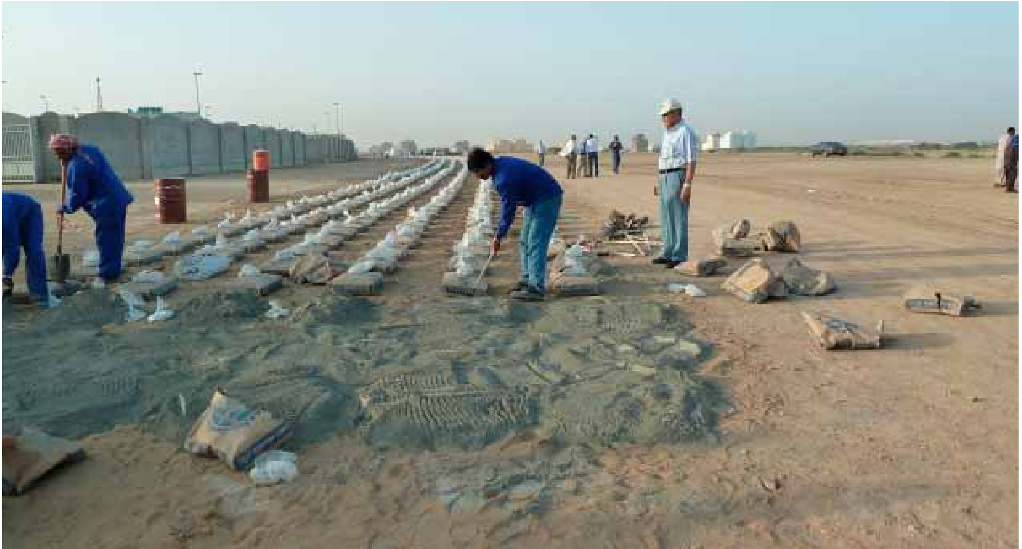
Manually distribution of the cement/NovoCrete
