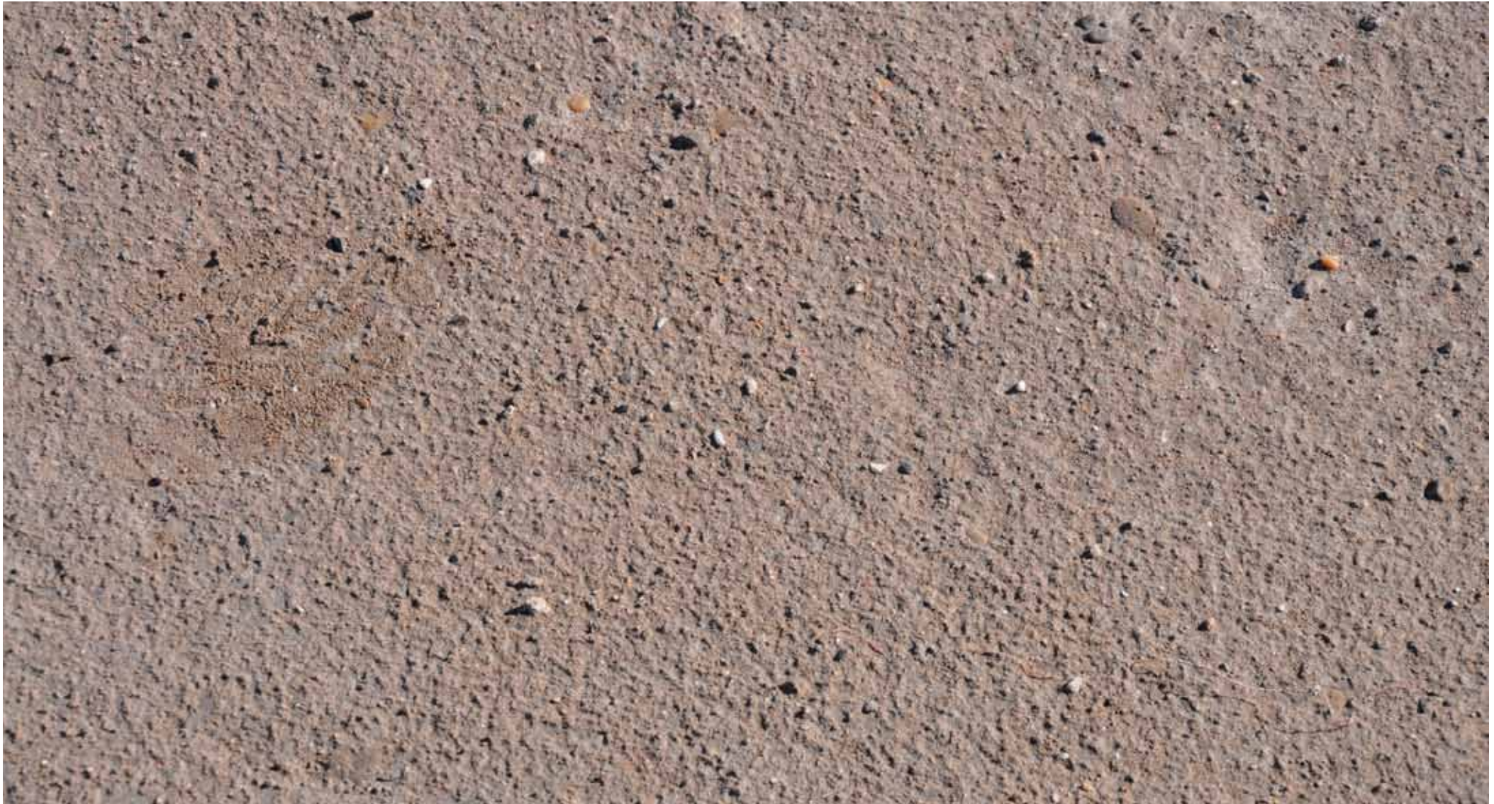
Stabilized area after one day - values in load bearing capacity > 300 \text{ MN/m}^2
