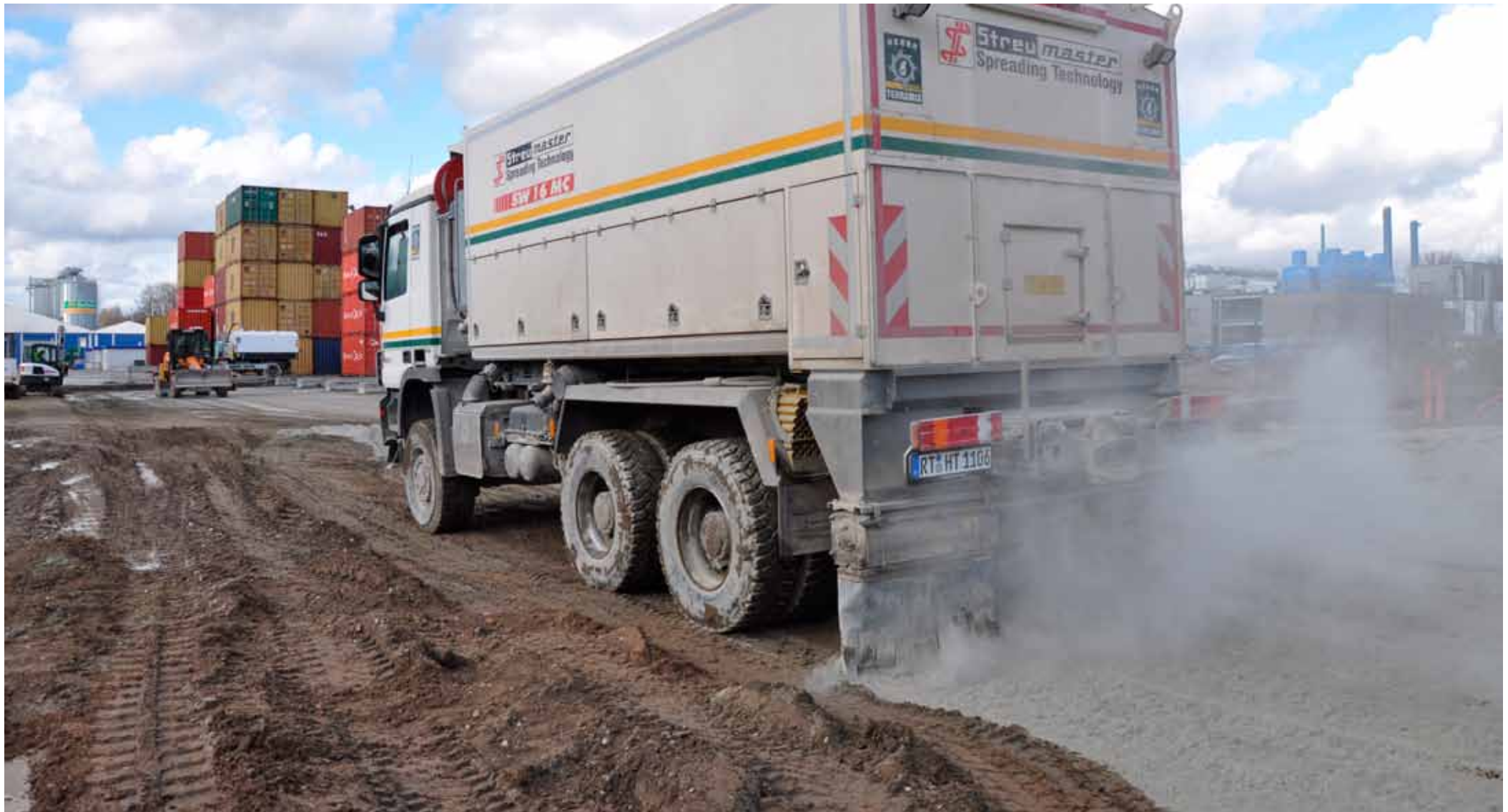
Spreading of the cement-Novocrete-mixture
