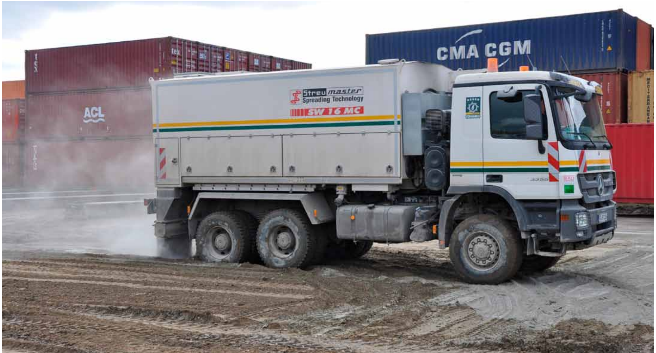
Spreading of the cement-Novocrete-mixture
