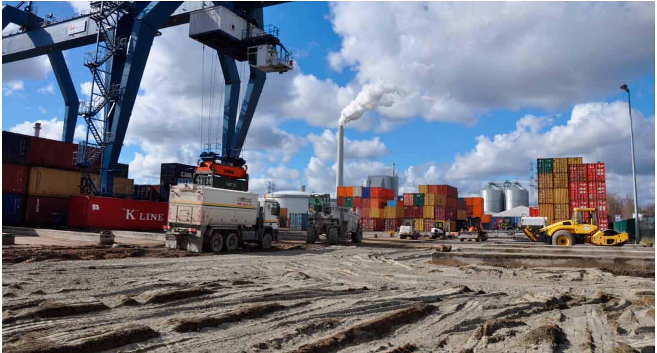
Spreading of the cement-Novocrete-mixture
