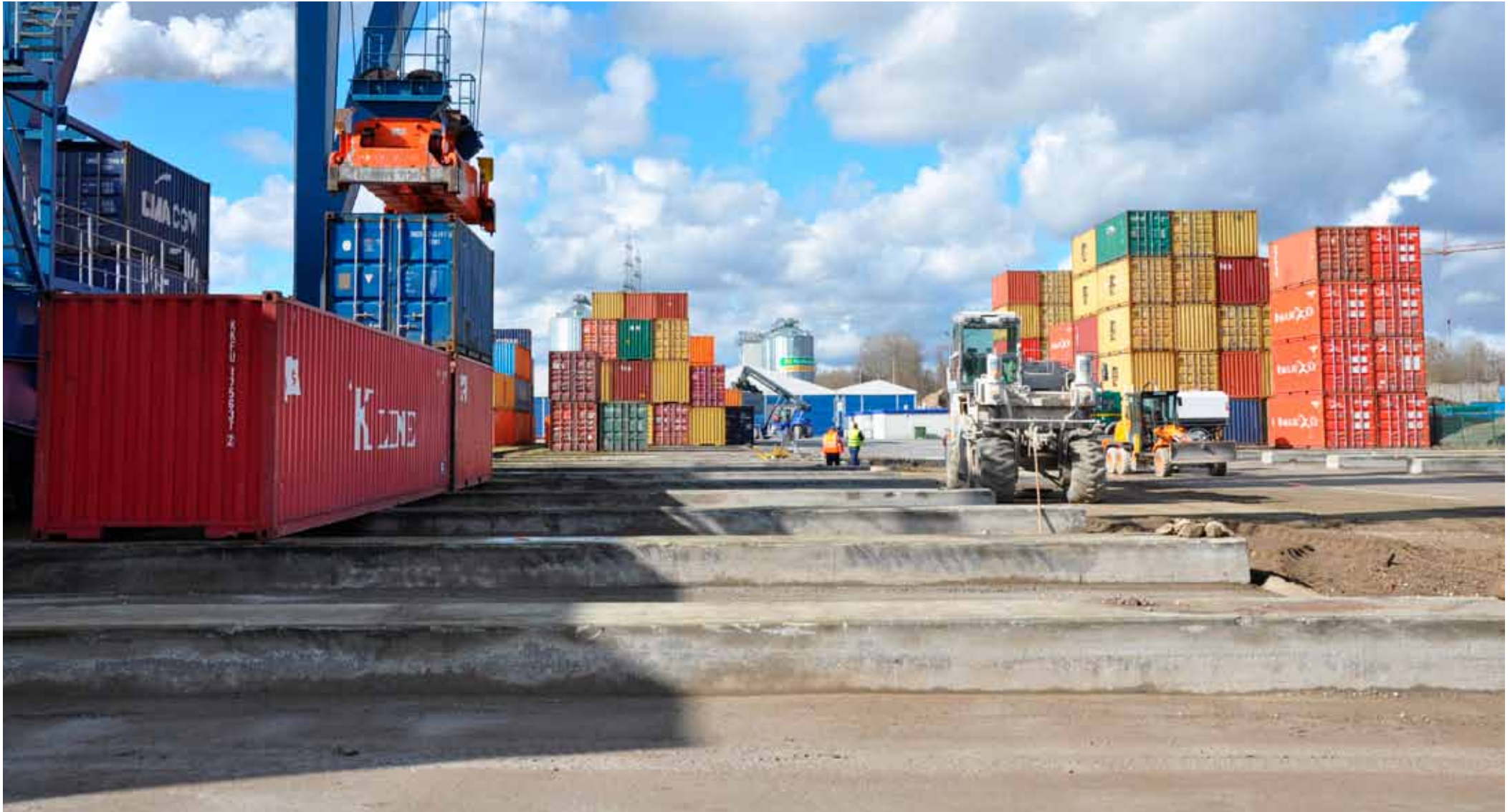
Stabilized area after one day - values in load bearing capacity > 300 \text{ MN/m}^2
