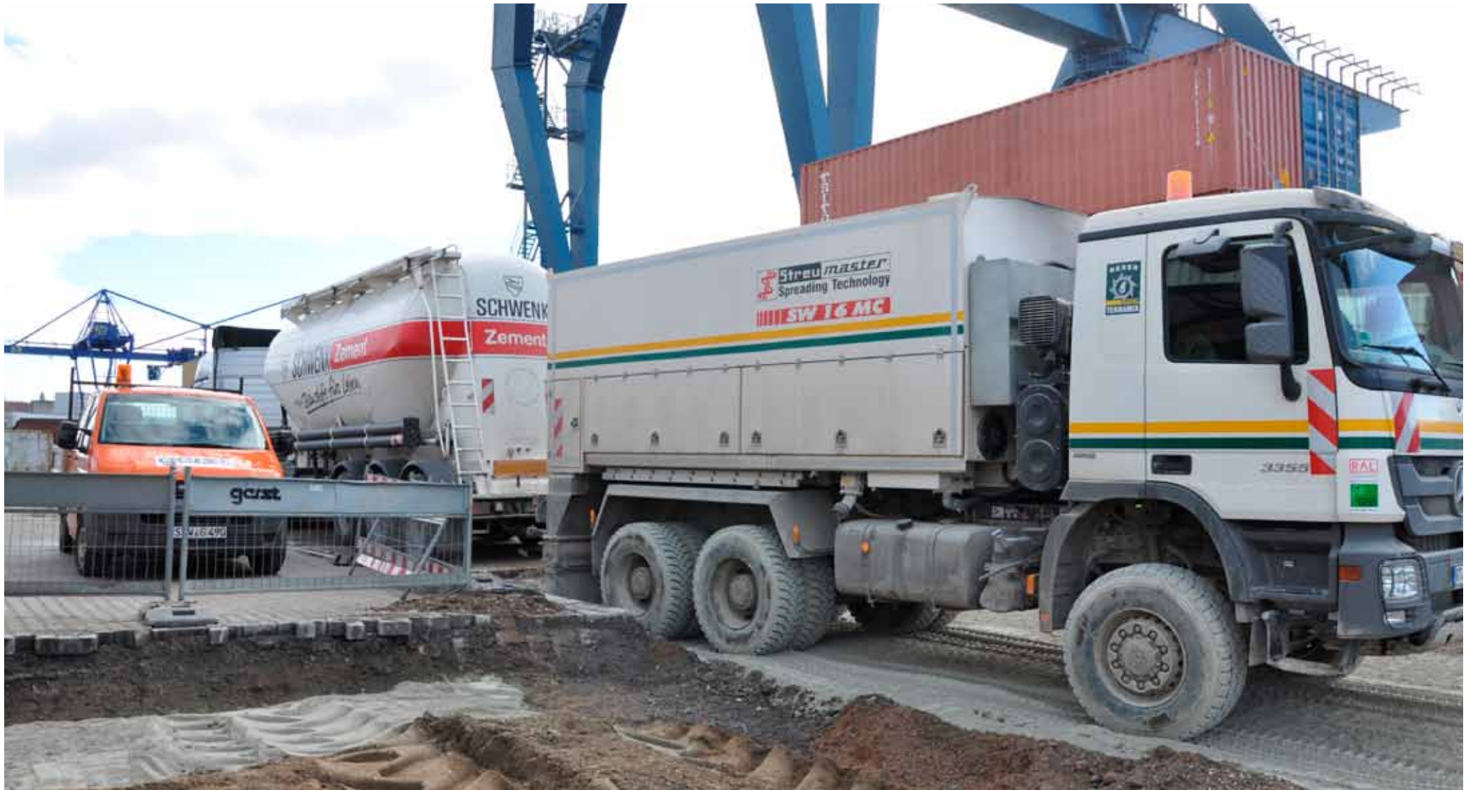
Loading of the spreading vehicle with the cement-Novocrete-mixture
