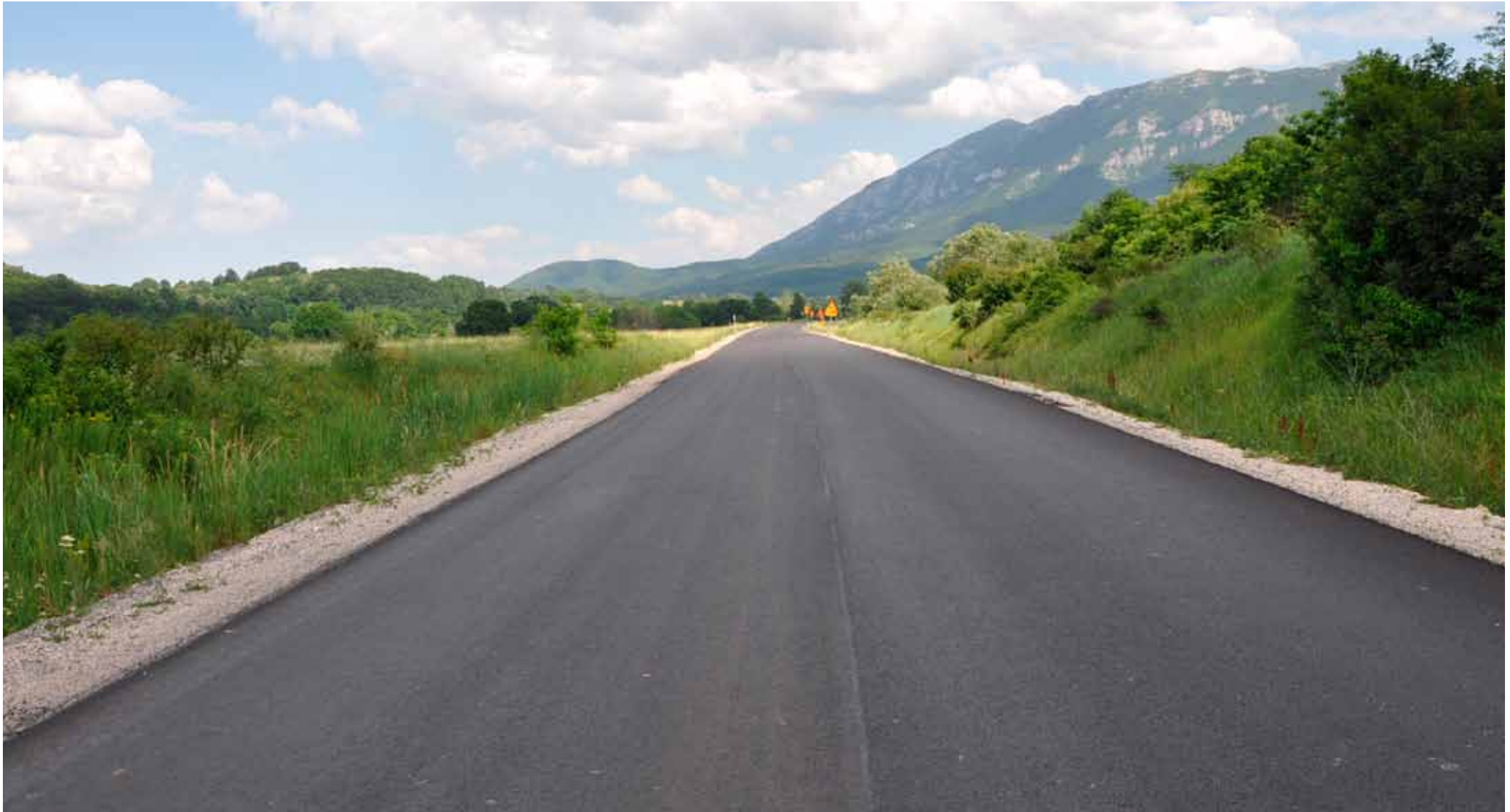
Road with new asphalt layer
