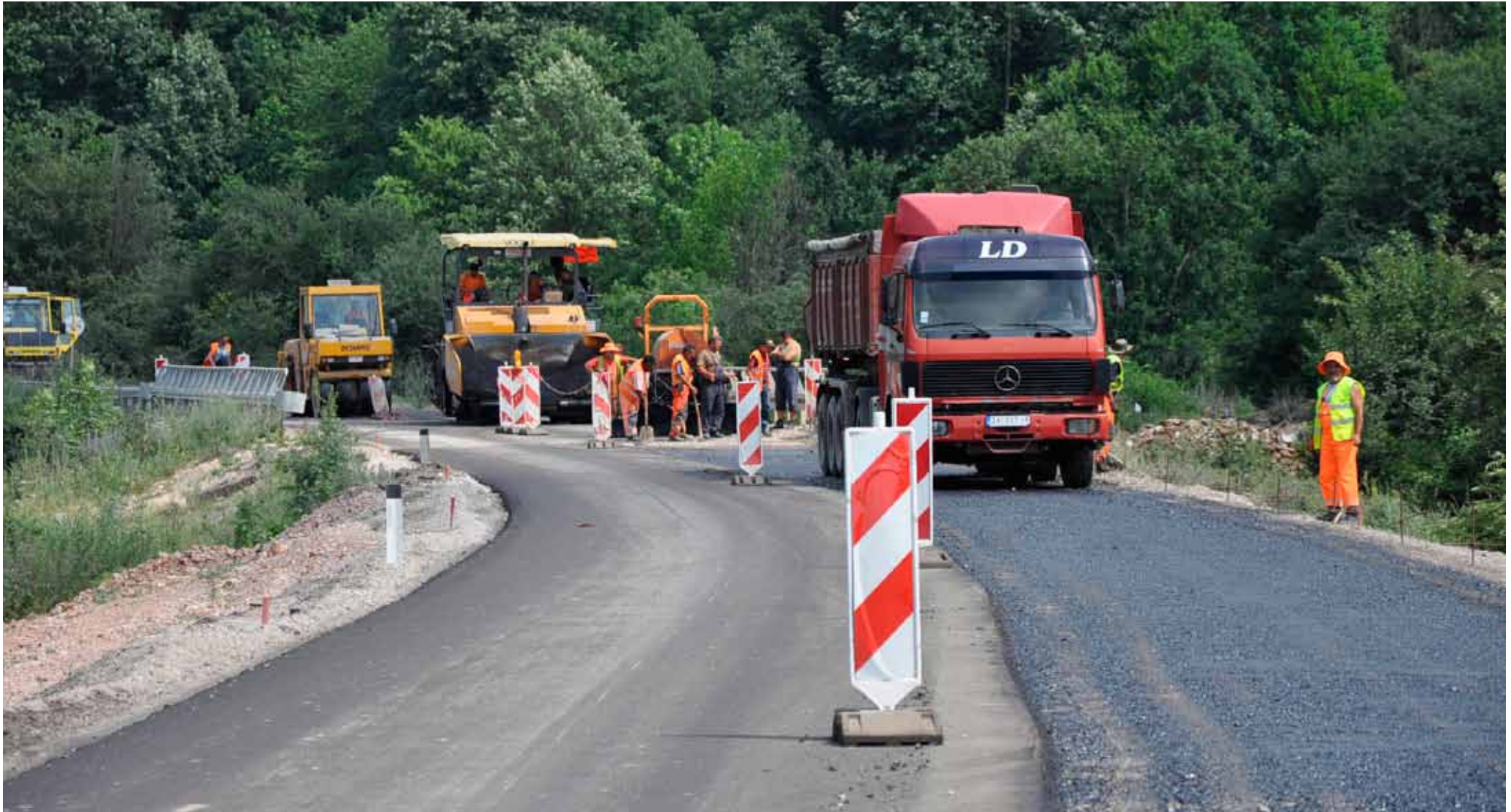
Fitting in of the new asphalt layer
