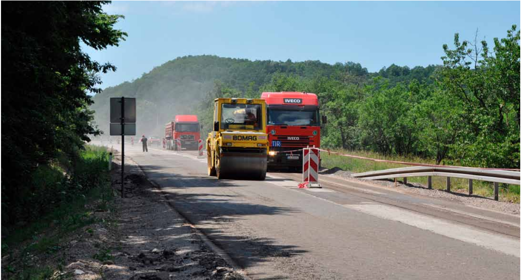
Compaction of the area
