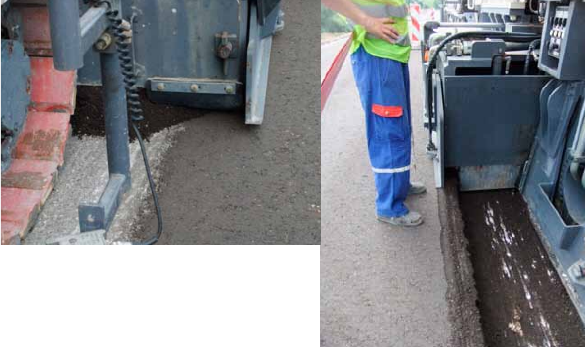
Use of the Mix Paver
