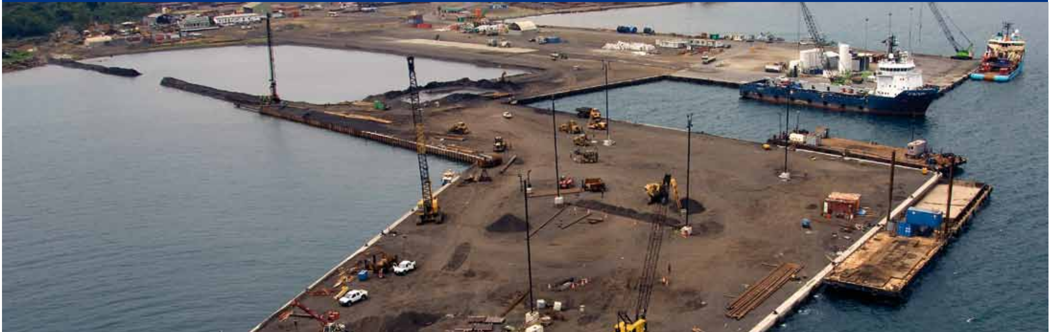
Construction of harbour facilities with NovoCrete®
