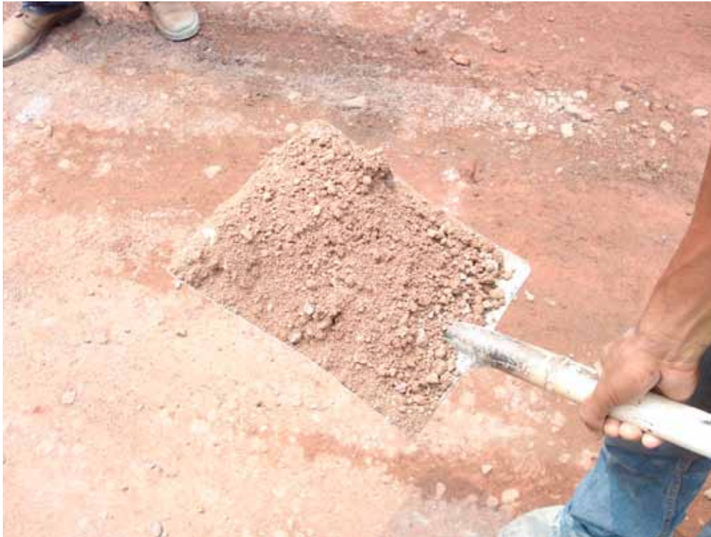
Fig 6: Homogenised NovoCrete® cement/soil mixture before compaction.
