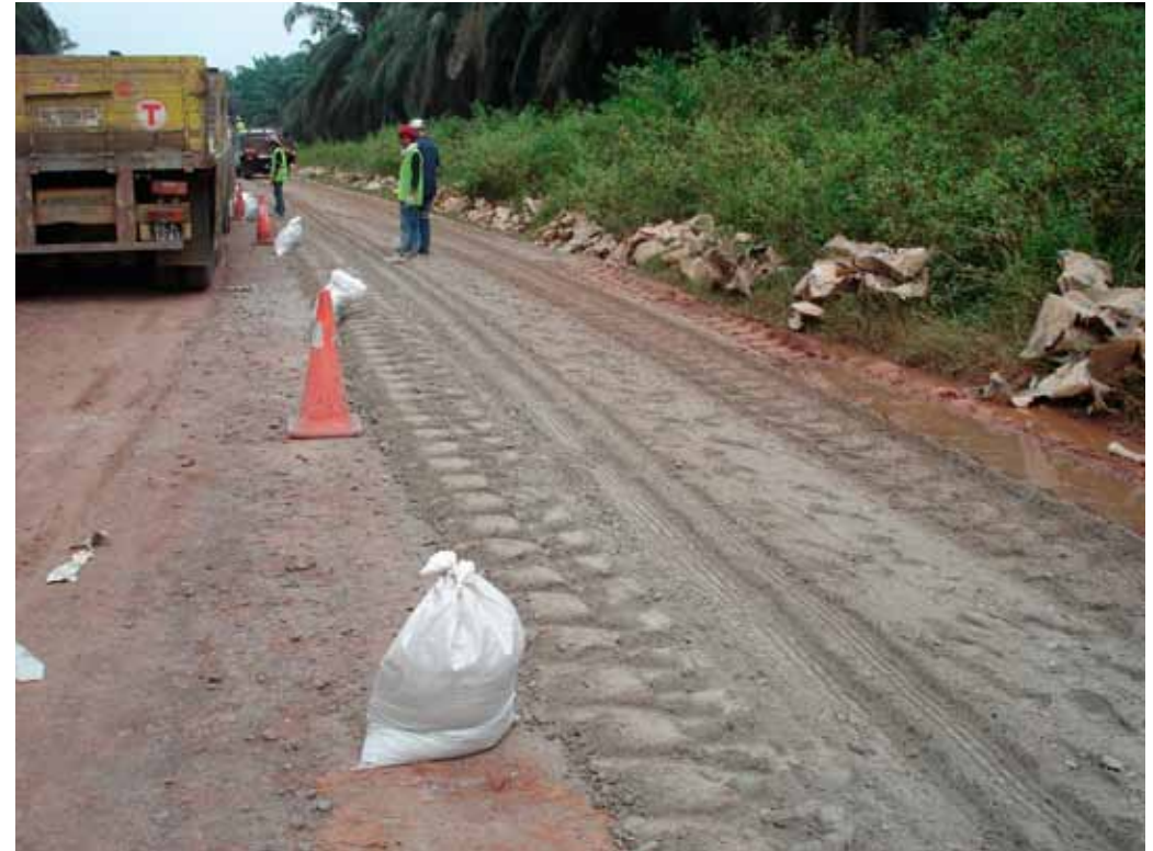
Fig 3: Laying the NovoCrete® ST additive.
