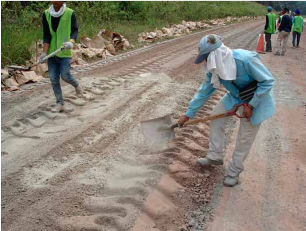
Fig 4: Manual distribution of the NovoCrete® ST additive over the spread cement.
