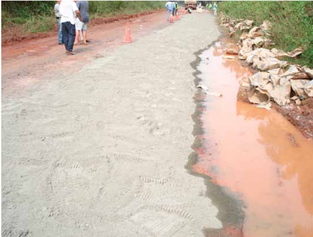
Fig 2: Spreading the cement supplied in bags of 50kg (CEM I 32.5 R).
