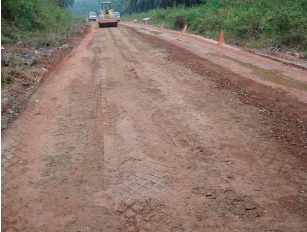
Fig 8: Dynamic compaction of the NovoCrete® base course with a smooth roller.
