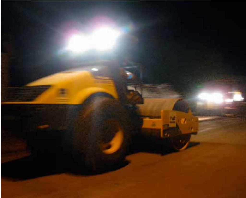
Static and dynamic compaction
