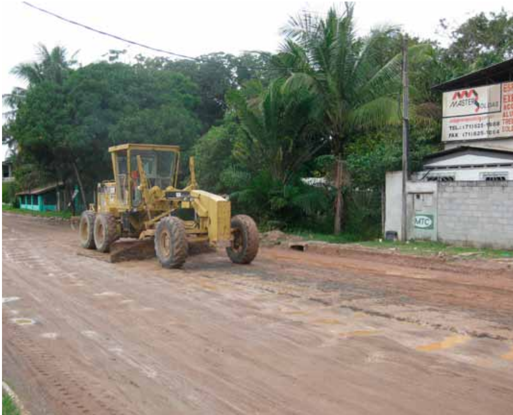
Use of a Grader for the levelling
