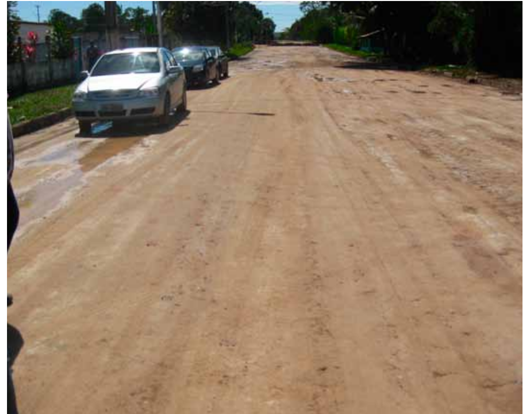
Area after compaction
