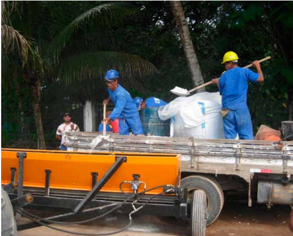
Filling of the spreading unit with the cement additive NovoCrete®
