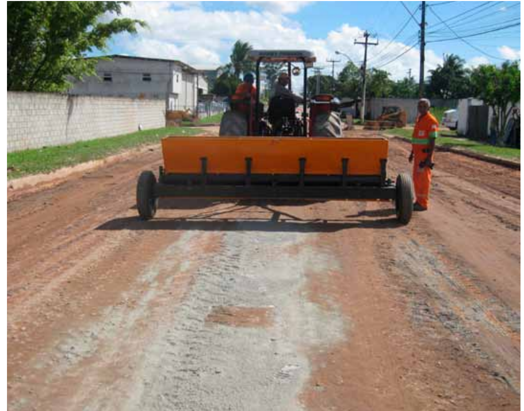
Tractor with the attached spreading unit for the cement additive NovoCrete®
