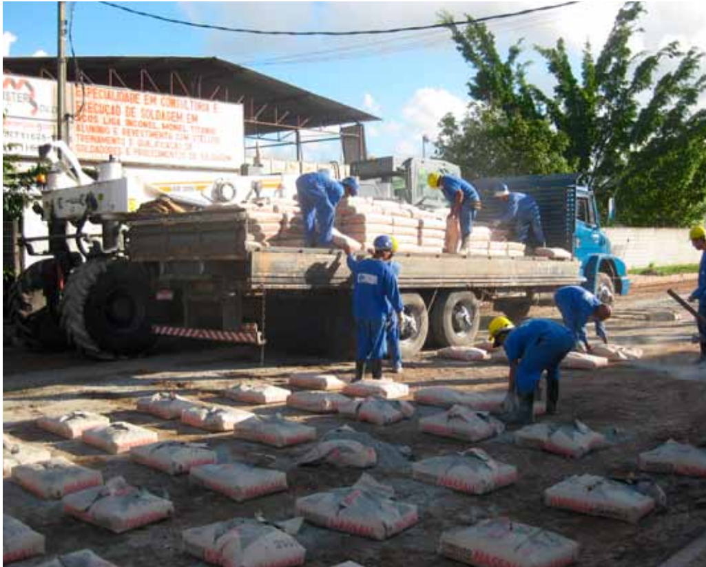
Delivery of the cement
