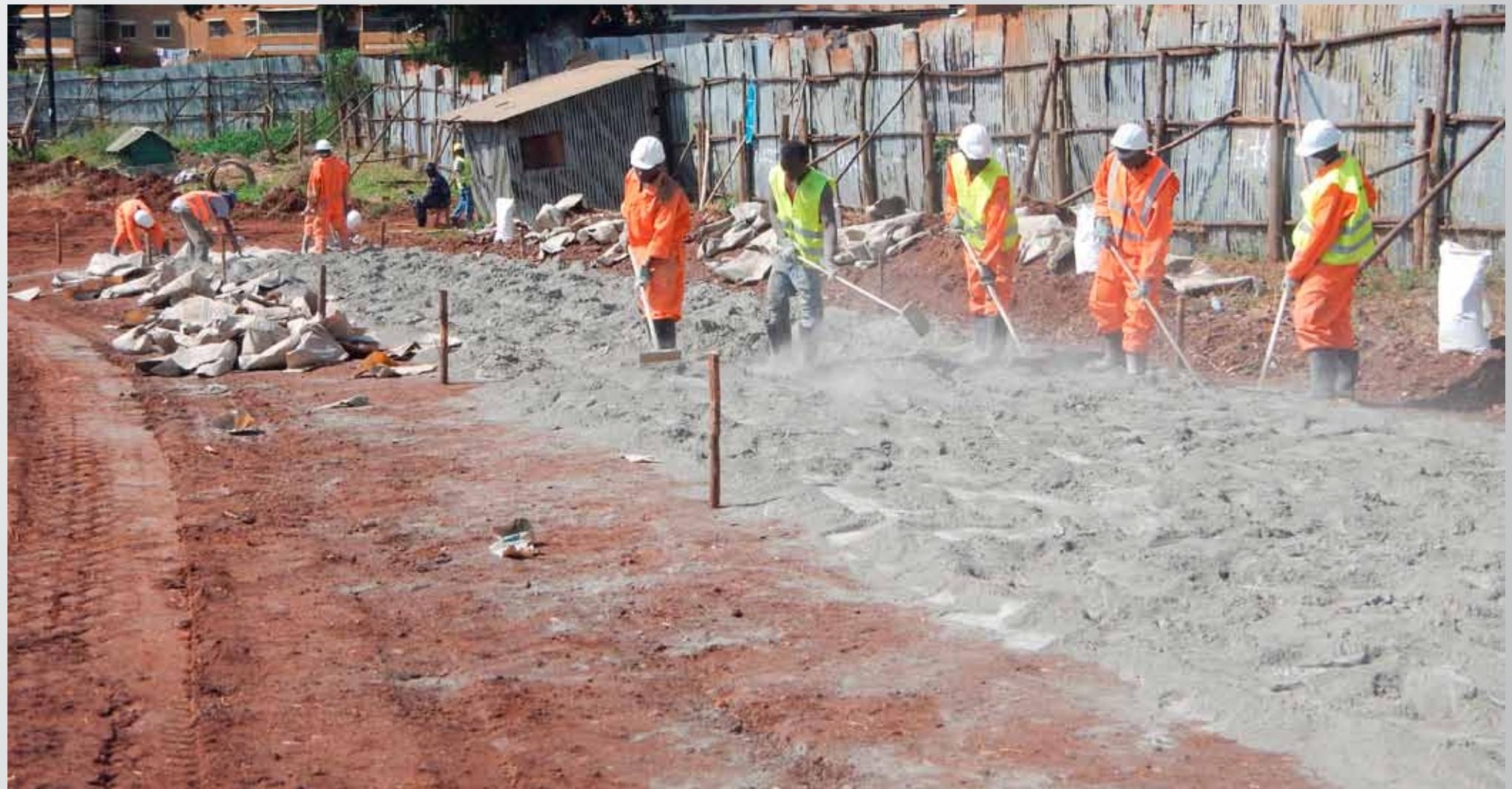
**Manually spreading of the exactly defined amount of NovoCrete® per m<sup>2</sup>**
