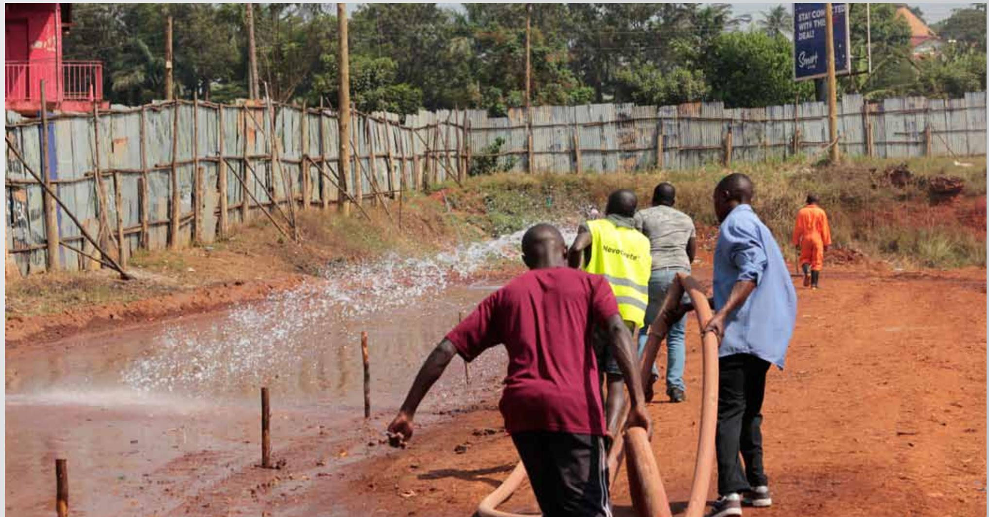
**Area after irrigation (protection against evaporation)**
