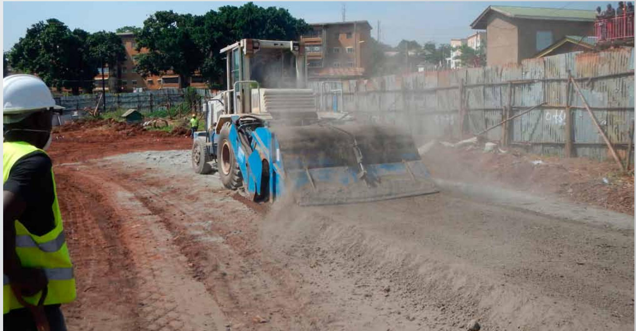
**Milling of the cement/NovoCrete® mixture to a milling depth of up to 0,3 m**
